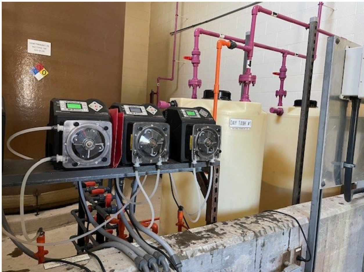
Figure 5.18 – Peristaltic Pump Chemical Feed
