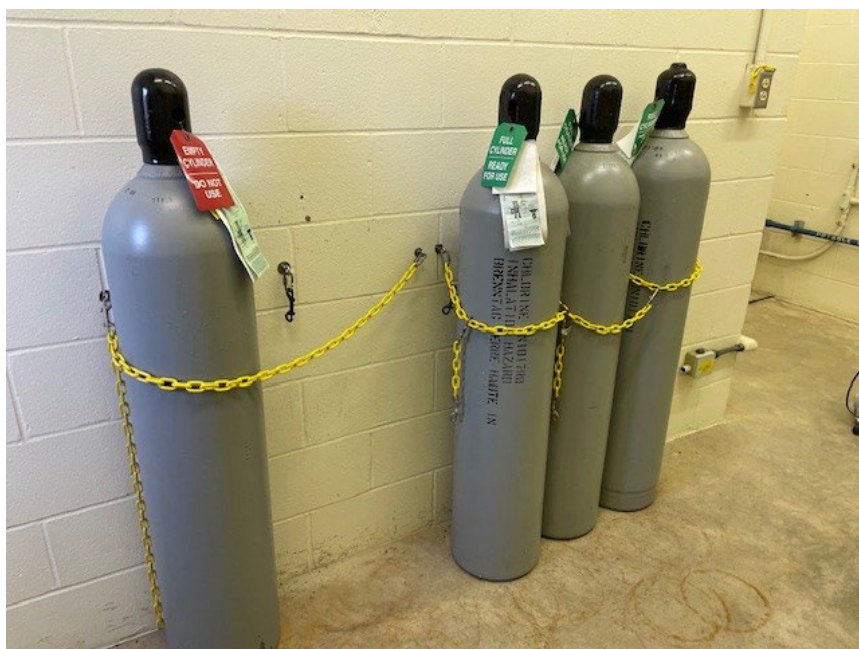
Figure 5.3 – Chlorine Cylinder Storage
