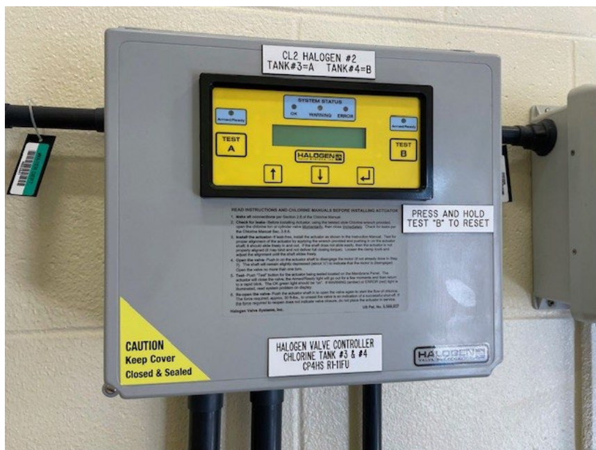
Figure 5.6 – Chlorine Valve Controller
