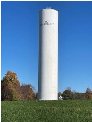
Figure 6.10 – Standpipe Tank
