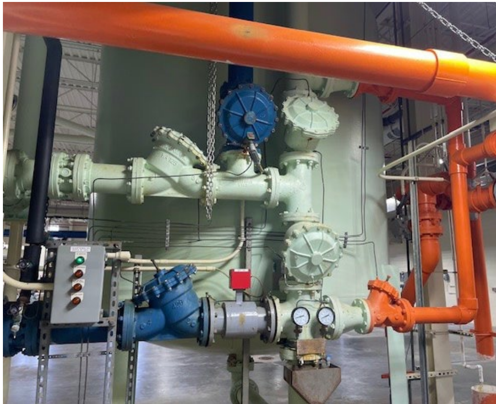
Figure 4.10 – Control Panel, Valves, and Pipes of a Softening Unit
