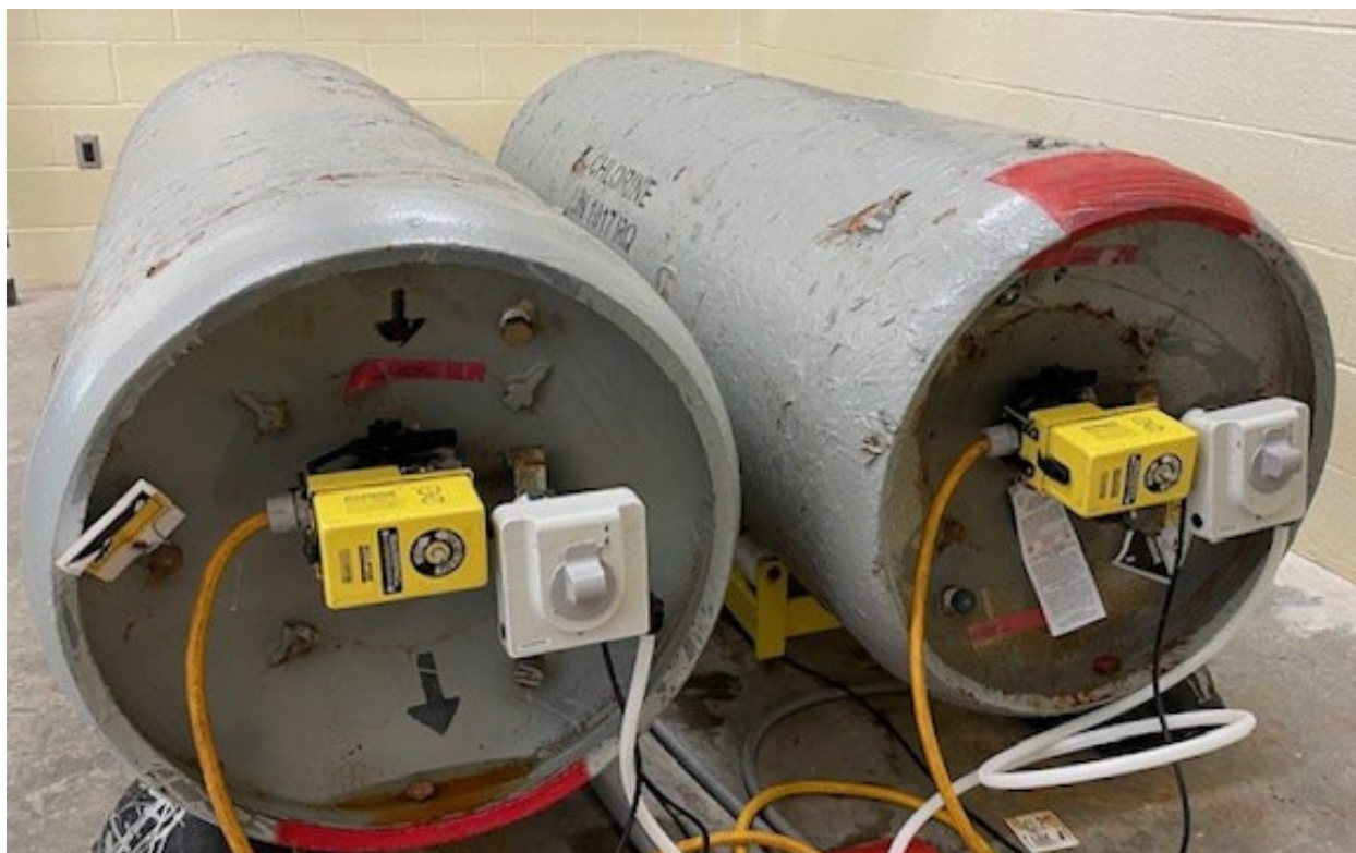
Figure 5.5 – Ton Container with Safety Valve Shutoff Actuator
