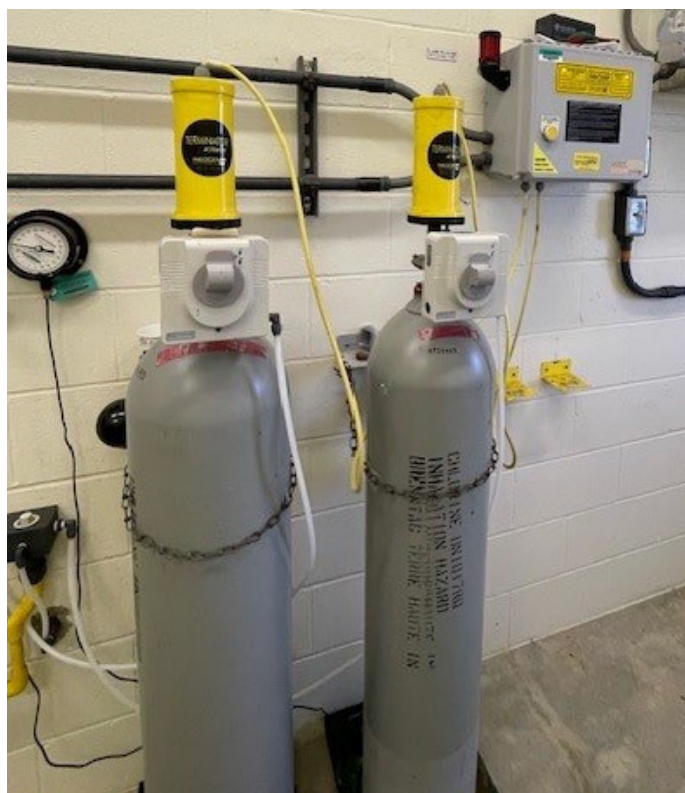
Figure 5.2 – 150lb Chlorine Cylinders and Chlorinator
