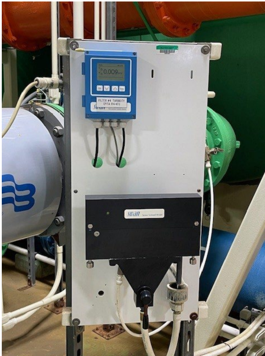
Figure 6.4 – Turbidimeter
