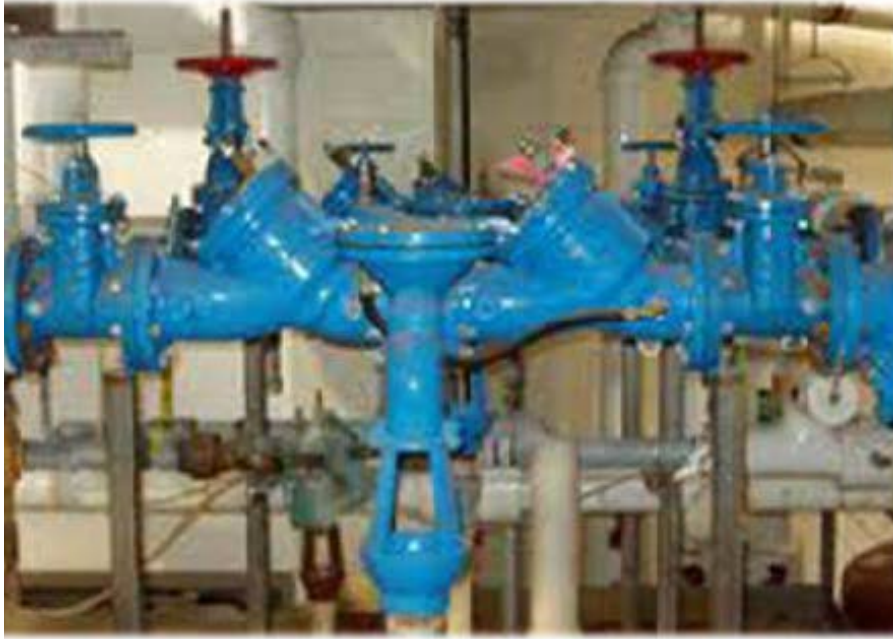
Figure 7.11– Reduced Pressure Principle Assembly Photo
