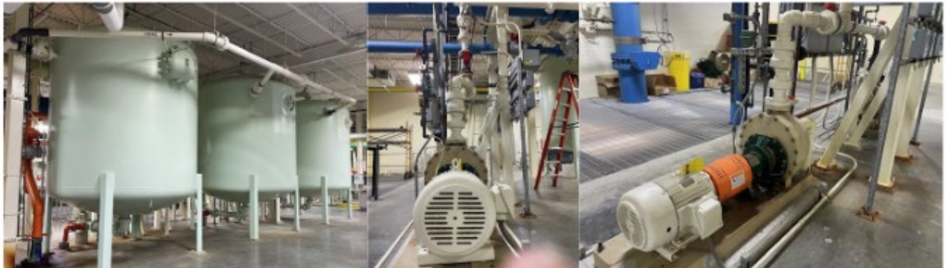
Figure 4.9 – Fiberglass Softening Tanks, Pump, and Pipes
