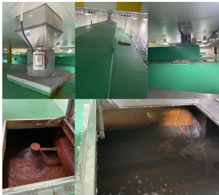
Figure 4.13 – Combination Aerator/Filtration Unit Components
