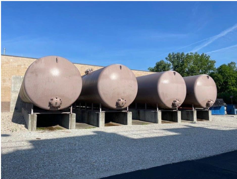
Figure 6.5 – Pressure Filters
