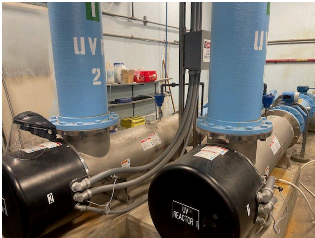
Figure 5.14 – UV Reactor
