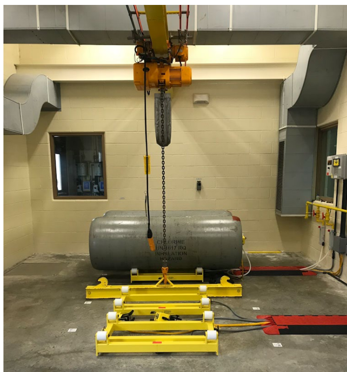
Figure 5.1 – One-Ton Chlorine Container
