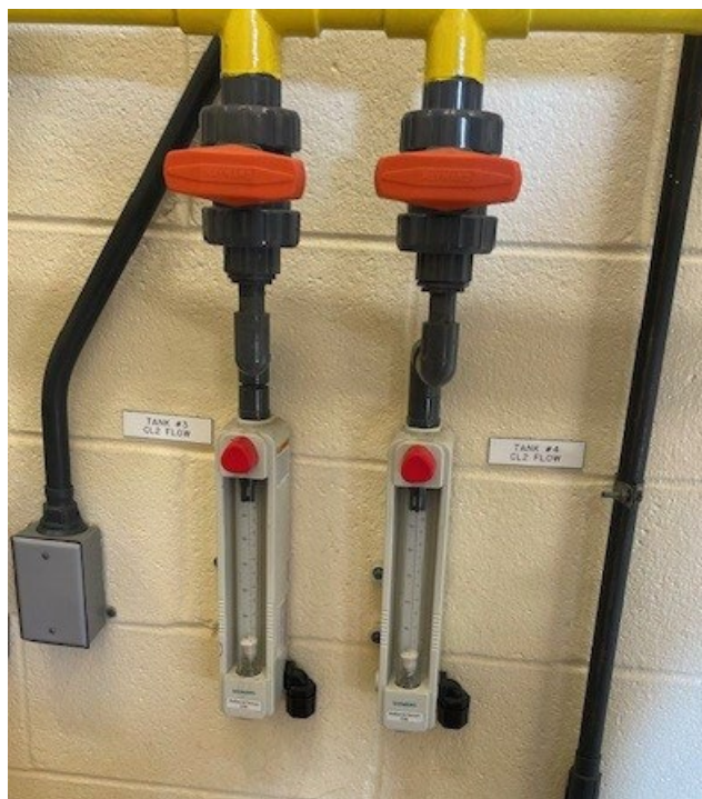
Figure 5.8 – Rotameter
