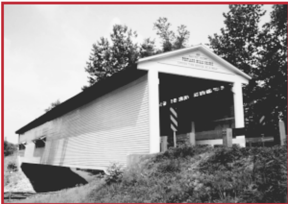
Portland Mills Covered Bridge, Parke County, built in 1856 by Henry Wolf with a Burr arch truss. It was restored in August 1996 and reopened to traffic with a thirteen ton limit. (14-61-21)
