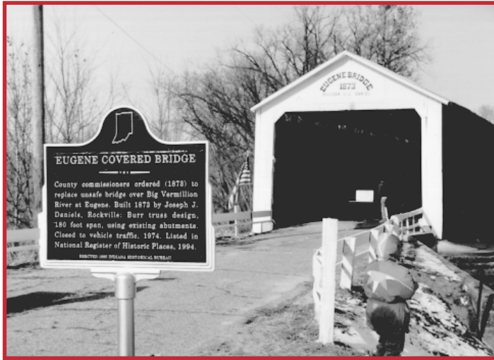
Eugene Covered Bridge, Vermillion County, built with a Burr arch truss. (14-83-05) Indiana Historical Marker number 83.1995.2.
