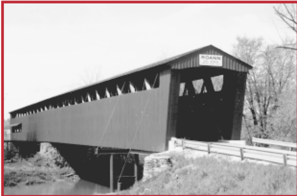
Roann Covered Bridge, Wabash County, was built in 1877 by the Smith Bridge Company with a Howe truss and restored in 1992. It is bypassed but open to traffic. (14-85-01)
