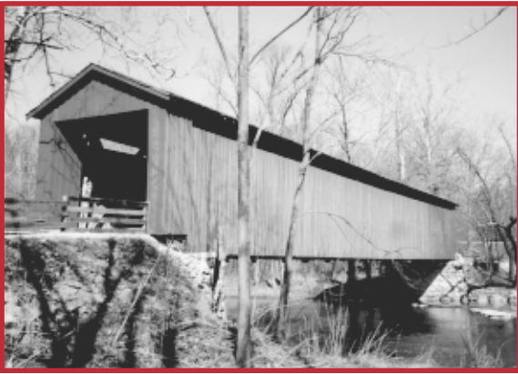
Cataract Falls Covered Bridge, Owen County, built in 1876 by Smith Bridge Company with a Smith type 4 truss. Restored in 1995 and closed to traffic. Located in Cataract Falls State Recreation Area. (14-60-01)
