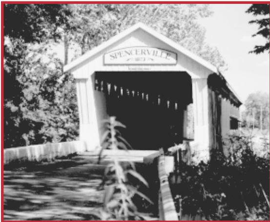
Spencerville Covered Bridge, De Kalb County, built in 1873 by John McKay with a Smith type 4 truss. Restored in 1990. (14-17-01)
