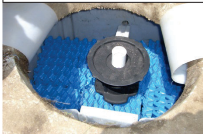
AIR LINE GLUED TO AIRLIFT COUPLING
