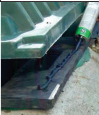
LINER & LID ARE SEALED TO TANK
