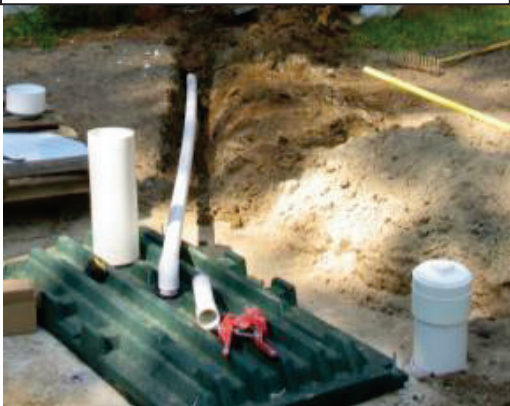
LINER & LID ARE SEALED TO TANK
