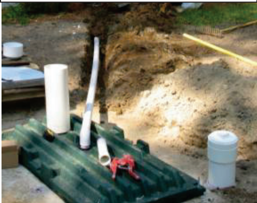
LINER & LID ARE SEALED TO TANK
