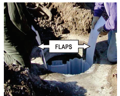
Step 3, 4, and 5: Outlet Pipe
