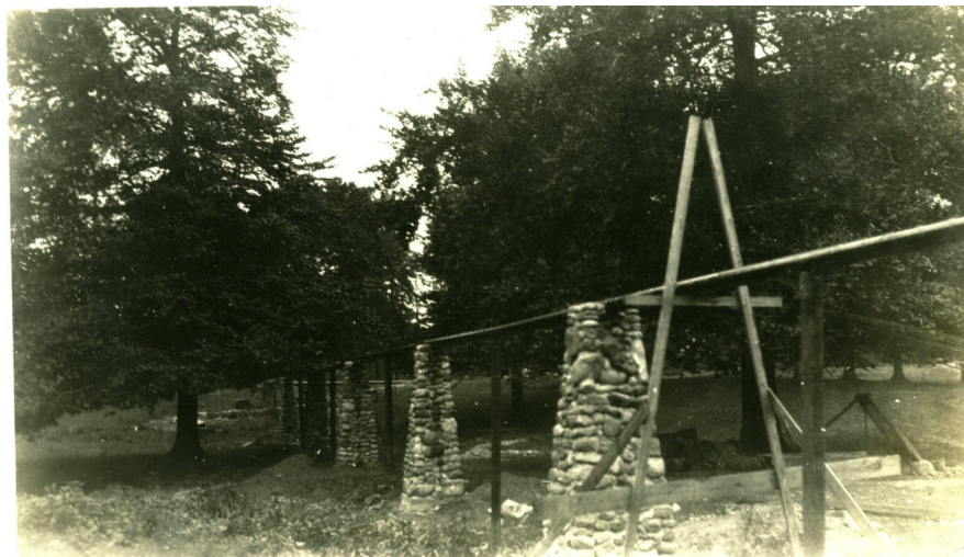
Water supply pipe line, Longcliff, Ind. Aug. 4, 1923
