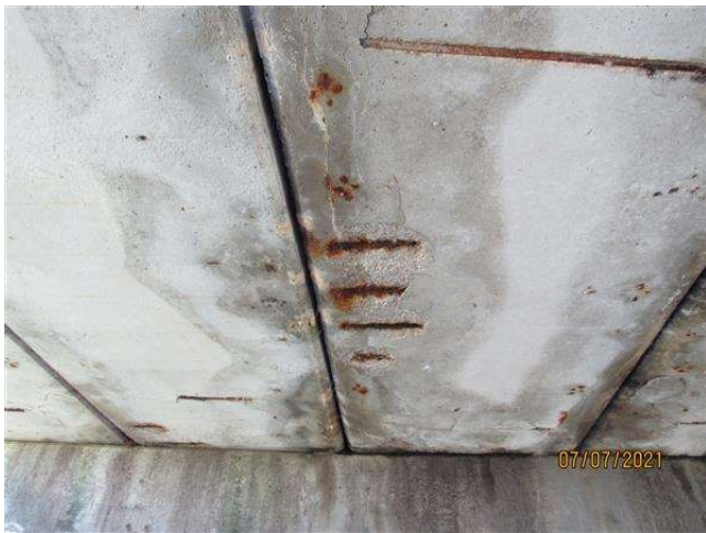
Exposing Steel in Beam 4
