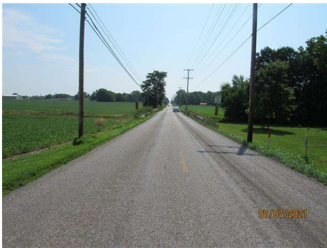
Alignment Looking East (20 Tons)
