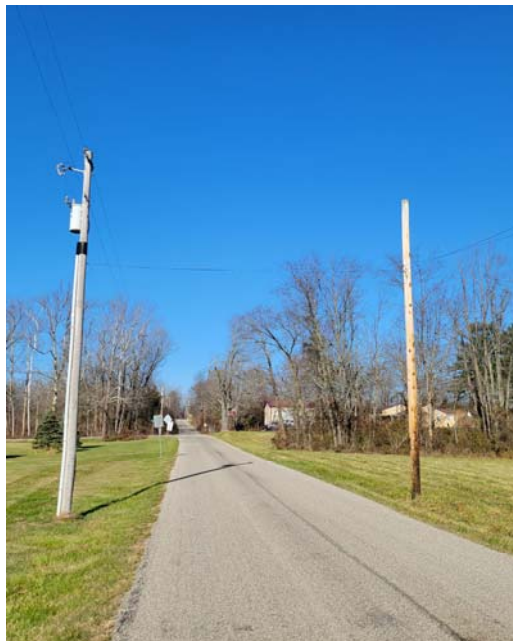
JC REMC Overhead (Left) North of Bridge 56
