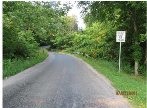
Alignment Looking South (15 Tons)
