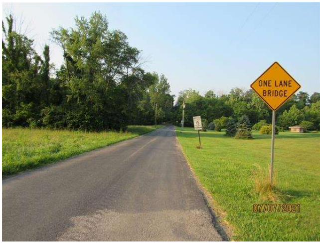
Alignment Looking South (15 Tons) (One Lane Bridge)
