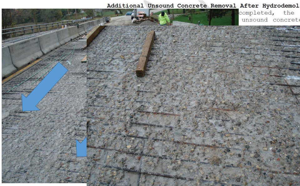
Additional Unsound Concrete Removal After Hydrodemolition
