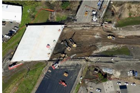
ODOT OR 213 over Washington St.
