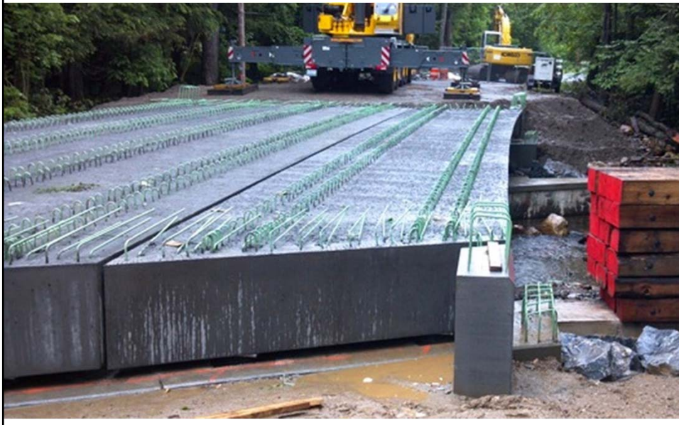
South Worthington, MA – Total Precast Built in 60 Days
