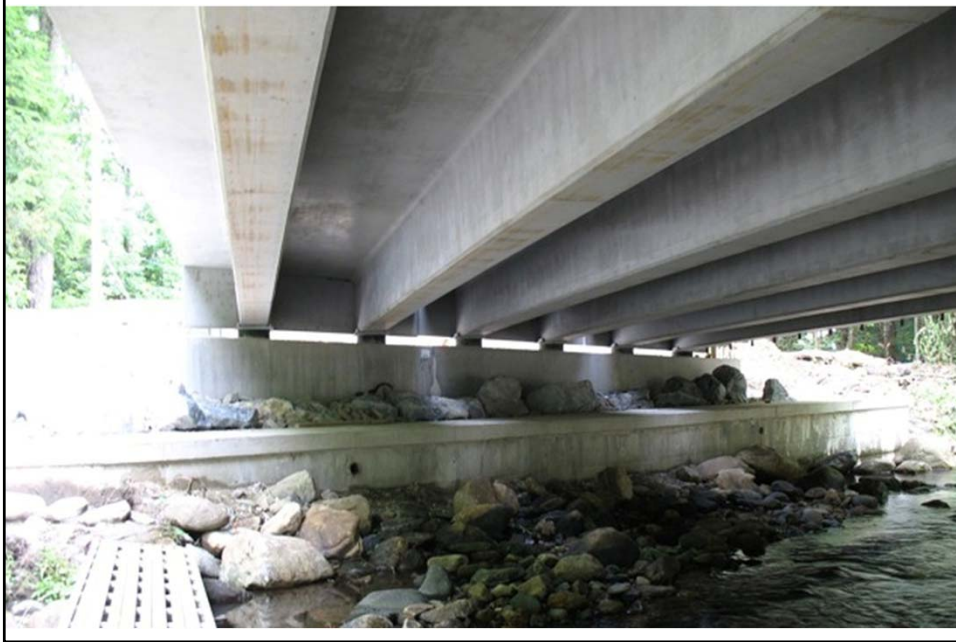
South Worthington, MA – Total Precast Built in 60 Days
