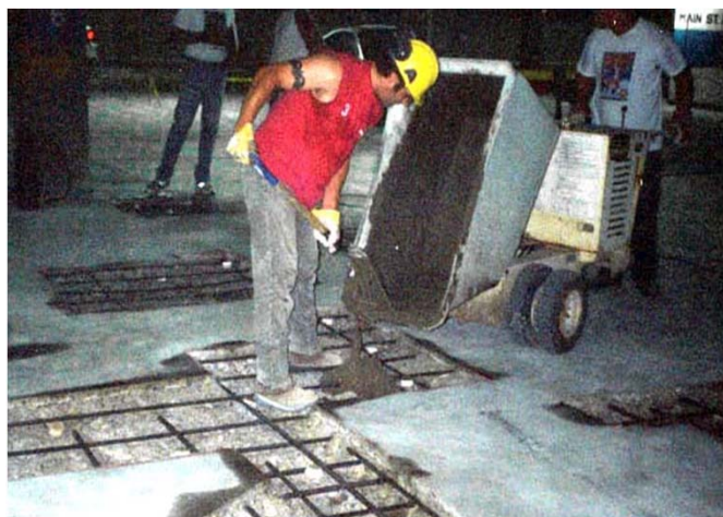
Embedding anodes with repair material.
