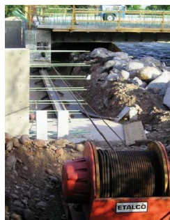
Pulling with strand jacks/ power winch
