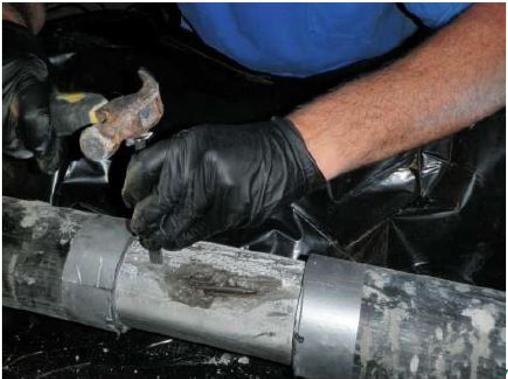
Chipping grout to expose strands and observe the level of saturation
