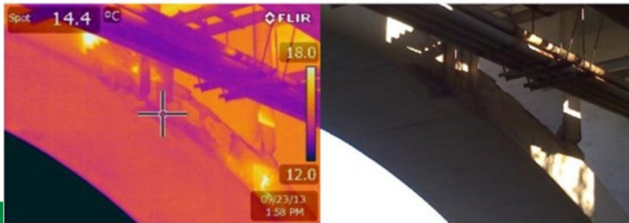
Figure 2: Upstream: Arch Spalling under Spandrel Columns A (left) and B (right)
