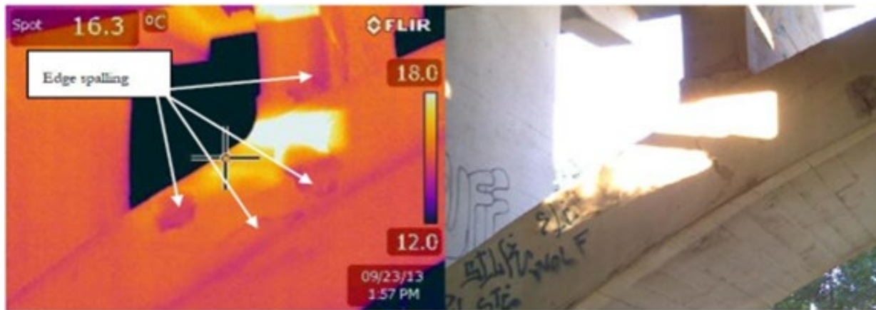
Figure 2: Upstream: Arch Spalling under Spandrel Columns A (left) and B (right)
