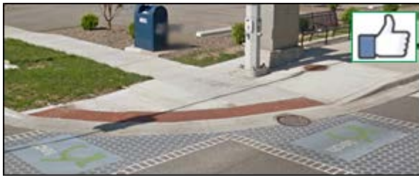
Detectable Warning Surface full width of the ramp.
