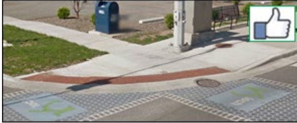
Detectable Warning Surface full width of the ramp.
