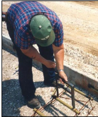
Figure 8.10.1 Dowel Bar Checker Device
