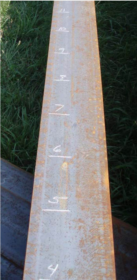
Figure 8. Steel H-Pile Marked in 1 ft Increments
