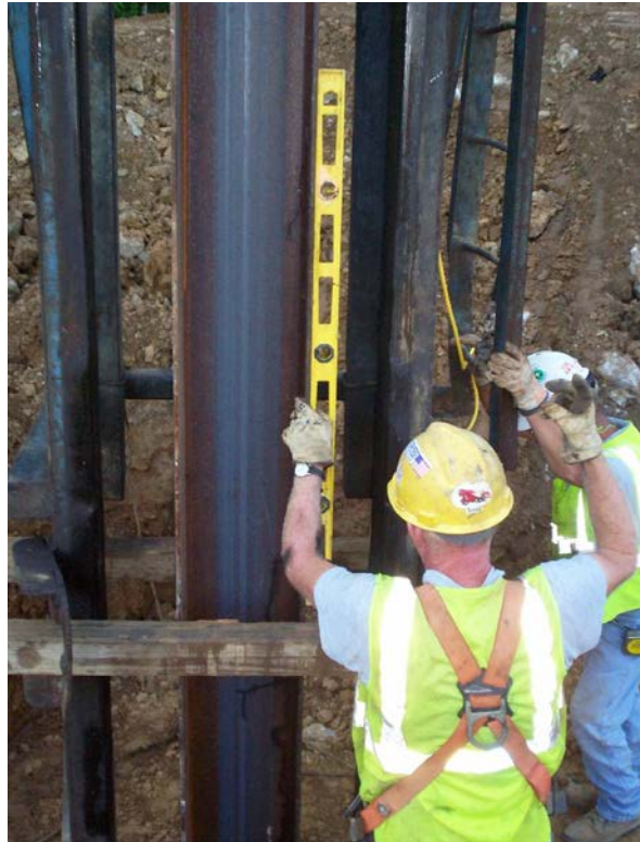
Figure 11 Checking Pile Alignment
