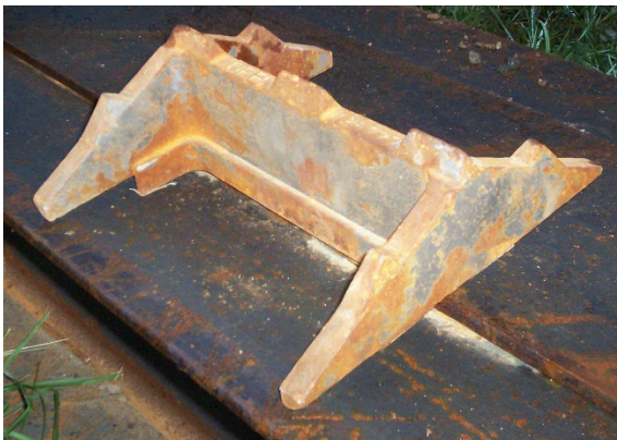
Figure 9 Bottom of H-Pile Shoe Tip
