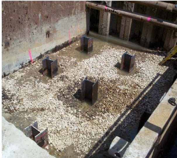
Figure 14. Piles cut-off at plan elevation
