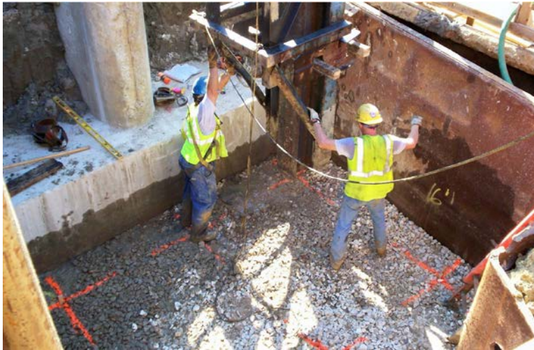
Figure 7. Pile Locations Marked at the Bottom of Footing
