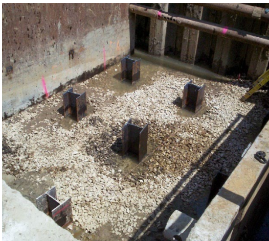
Figure 14. Piles cut-off at plan elevation
