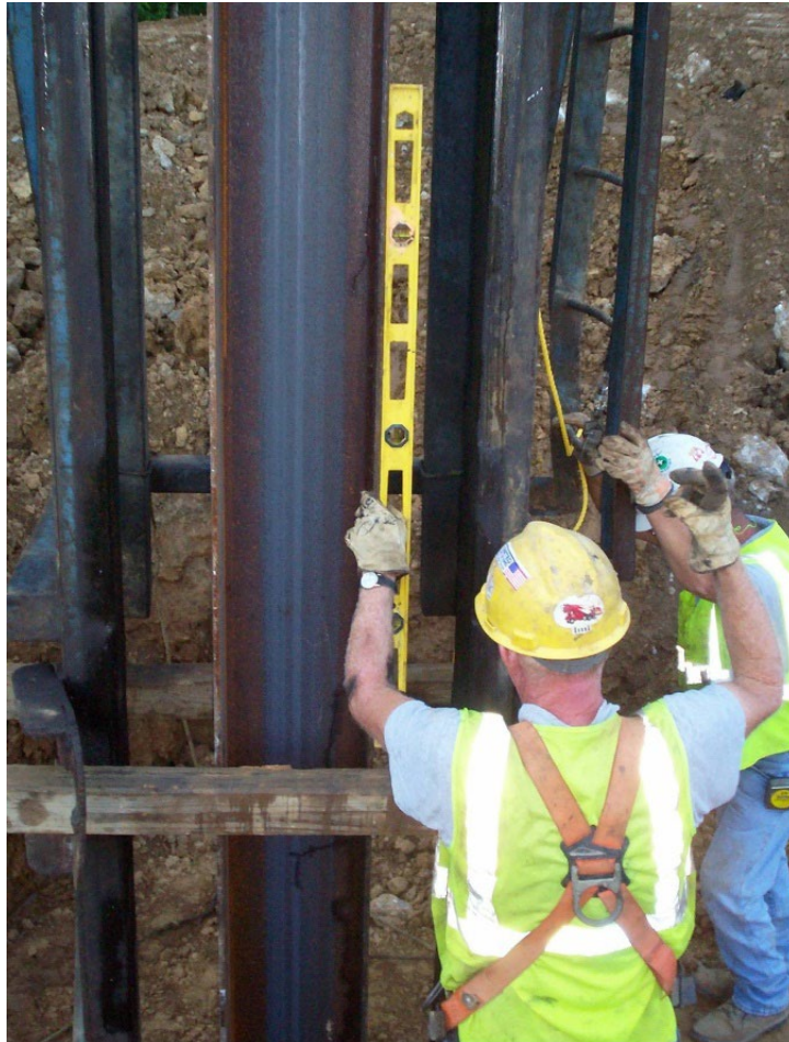
Figure 11 Contractor Checking Pile Alignment
