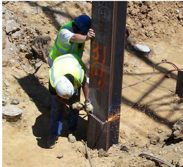
Figure 13. Pile being cut off at the plan elevation.
