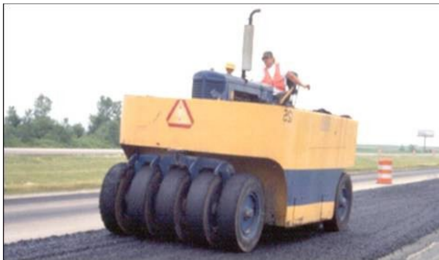
Figure 13.24-7. Pneumatic Tire Roller
