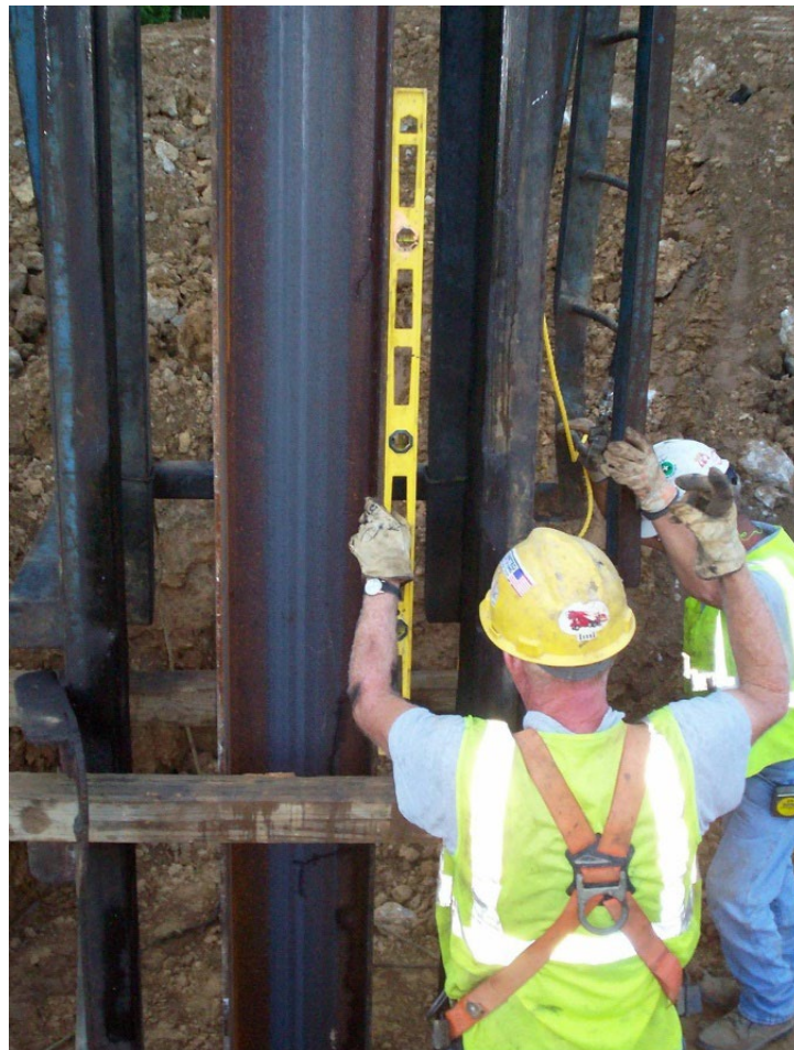
Figure 11. Contractor Checking Pile Alignment
