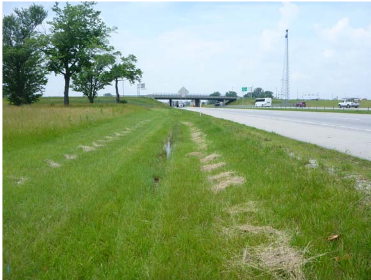
Photo 29: View of the southeast quadrant of the Campus Parkway Interchange (facing west; June 19, 2014).
