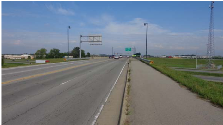
Photo 19: View of Campus Parkway Bridge over I-69 (facing northwest; September 4, 2014).
