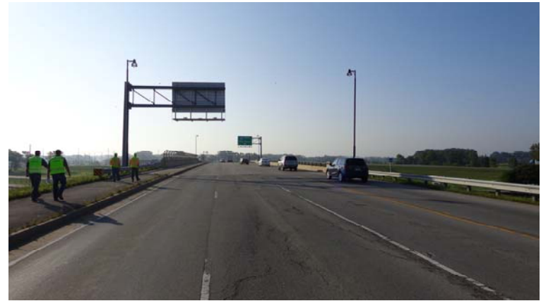
Photo 18: View of the Campus Parkway Bridge over I-69 (facing southeast; September 4, 2014)
