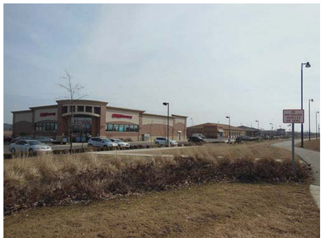
Campus Parkway and Corporate Parkway looking NE
