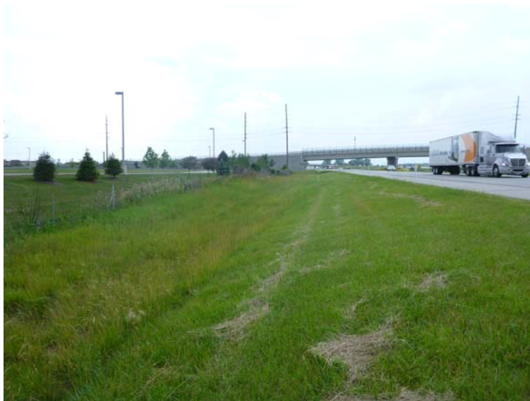
Photo 37: View of roadside drainage along I-69 near the project terminus (facing west; June 19, 2014). Note the Olio Road Overpass in the background.
