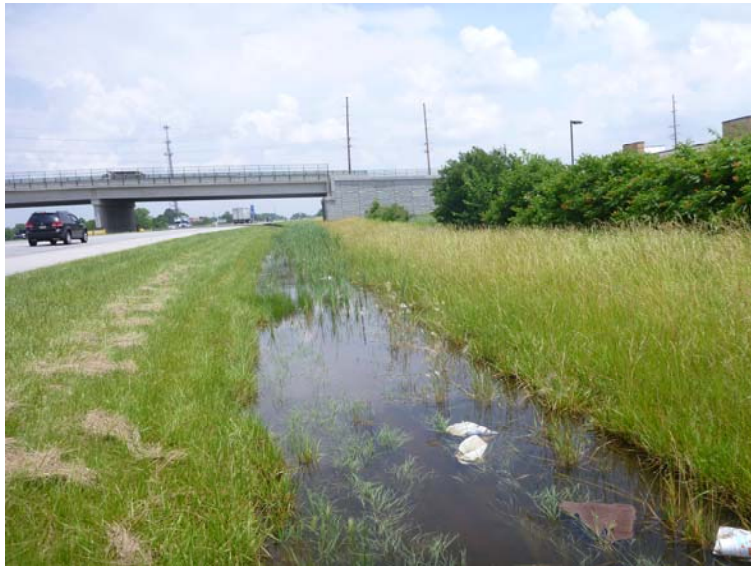
Photo 33: View of roadside drainage along the I-69 eastbound on-ramp (facing east; June 19, 2014). Note the wetland entirely contained within roadside drainage at this location.
