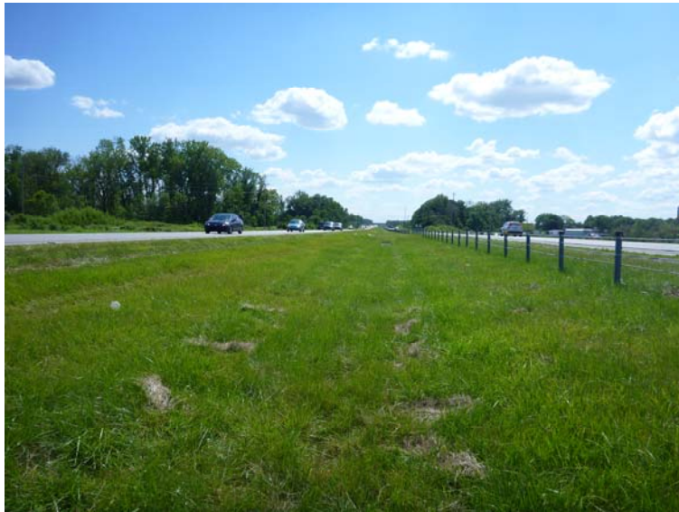
Photo 1: View of I-69 and its median near the project terminus (facing southwest; July 10, 2014).
