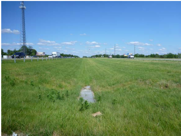
Photo 35: View of I-69 and its median (facing east; July 10, 2014).
