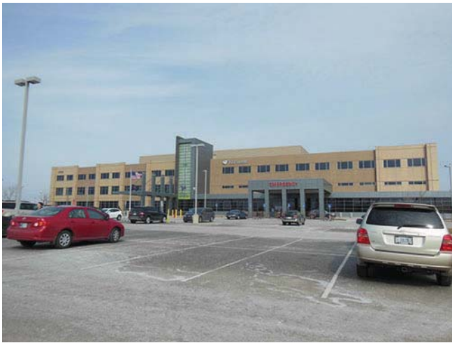
136th Street_13914 Southeastern Parkway looking N
