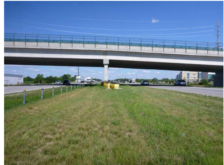
Photo 34: View of the Olio Road Overpass (facing east; July 10, 2014).
