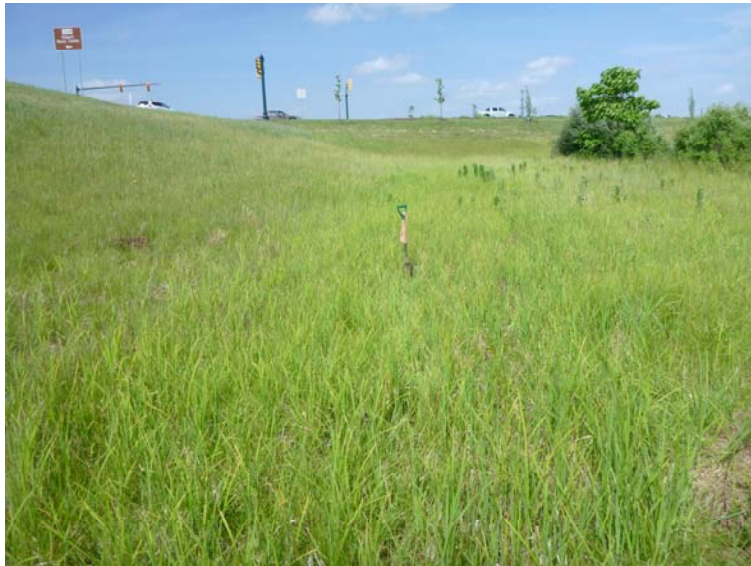
Photo 17: View of roadside drainage along the I-69 northbound off-ramp to Campus Parkway (facing northeast; June 17, 2014). Note the wetland entirely contained within the roadside drainage.
