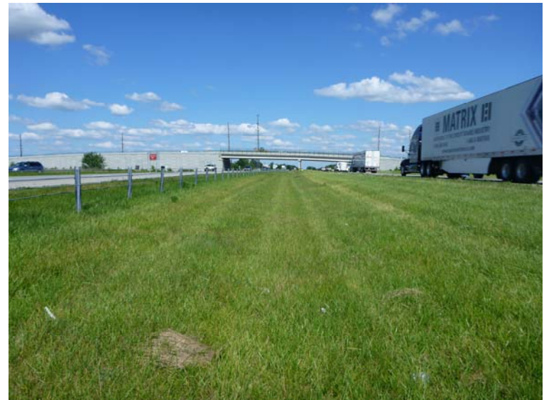
Photo 28: View of I-69 and its median (facing east; July 10, 2014). Note the Olio Road Overpass in the background.
