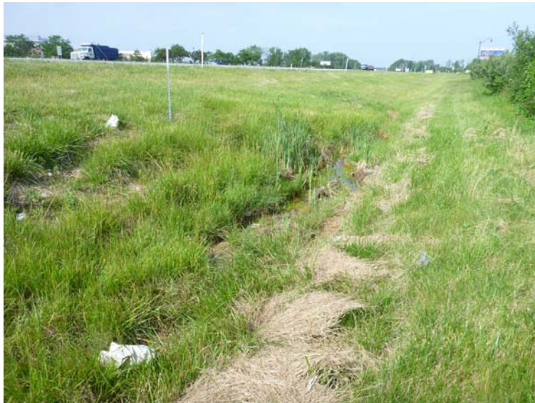
Photo 5: View of the roadside drainage along I-69 (facing southwest; June 18, 2014). Note the wetland entirely contained within the roadside drainage at this location.
