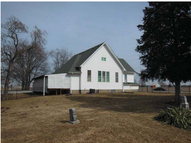
45005_Olio Road_Bethlehem Brethren Church and Cemetery looking NE
