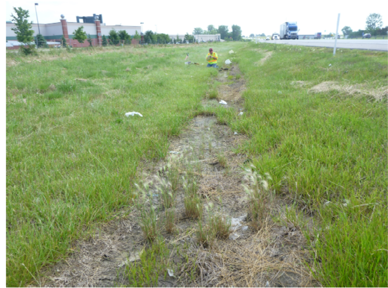
Photo 2: View of the roadside drainage along I-69 (facing northeast; June 18, 2014). Note the wetland entirely contained within the roadside drainage at this location.
