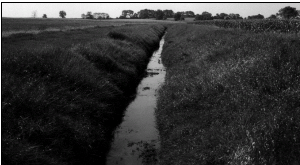
Exhibit 3.3a: Typical Example of a Man-Made Ditch with Grass Lining (Source: IDNR Files)
