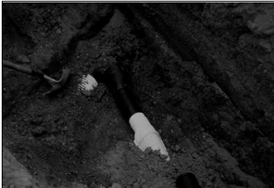
Exhibit 202a: Tile Drain Repair/Replacement (Source: NRCS Files)
