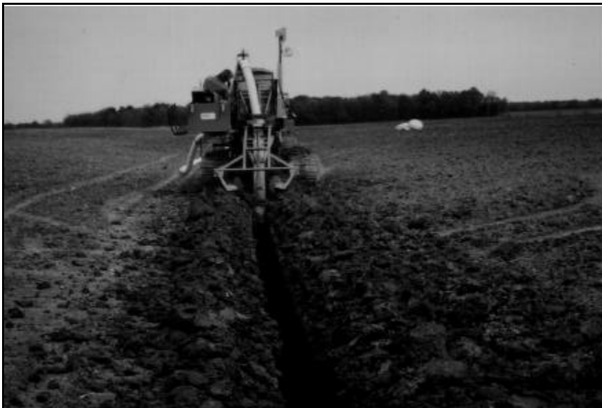
Exhibit 201a: Tile Drain Installation (Source: NRCS Files)
