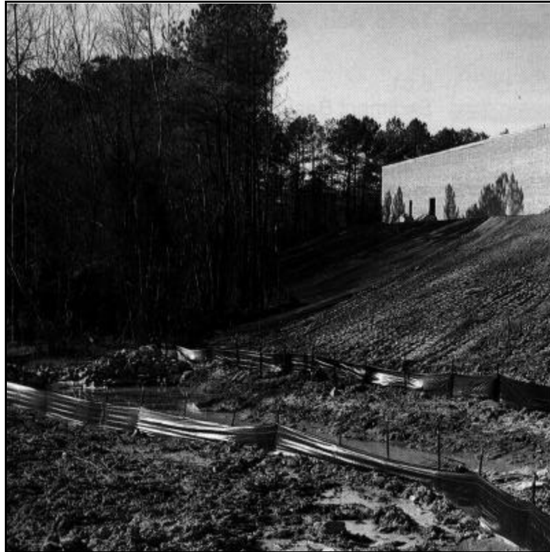
Exhibit 105a: Silt Fencing (Source: North Carolina Erosion Control Manual)
