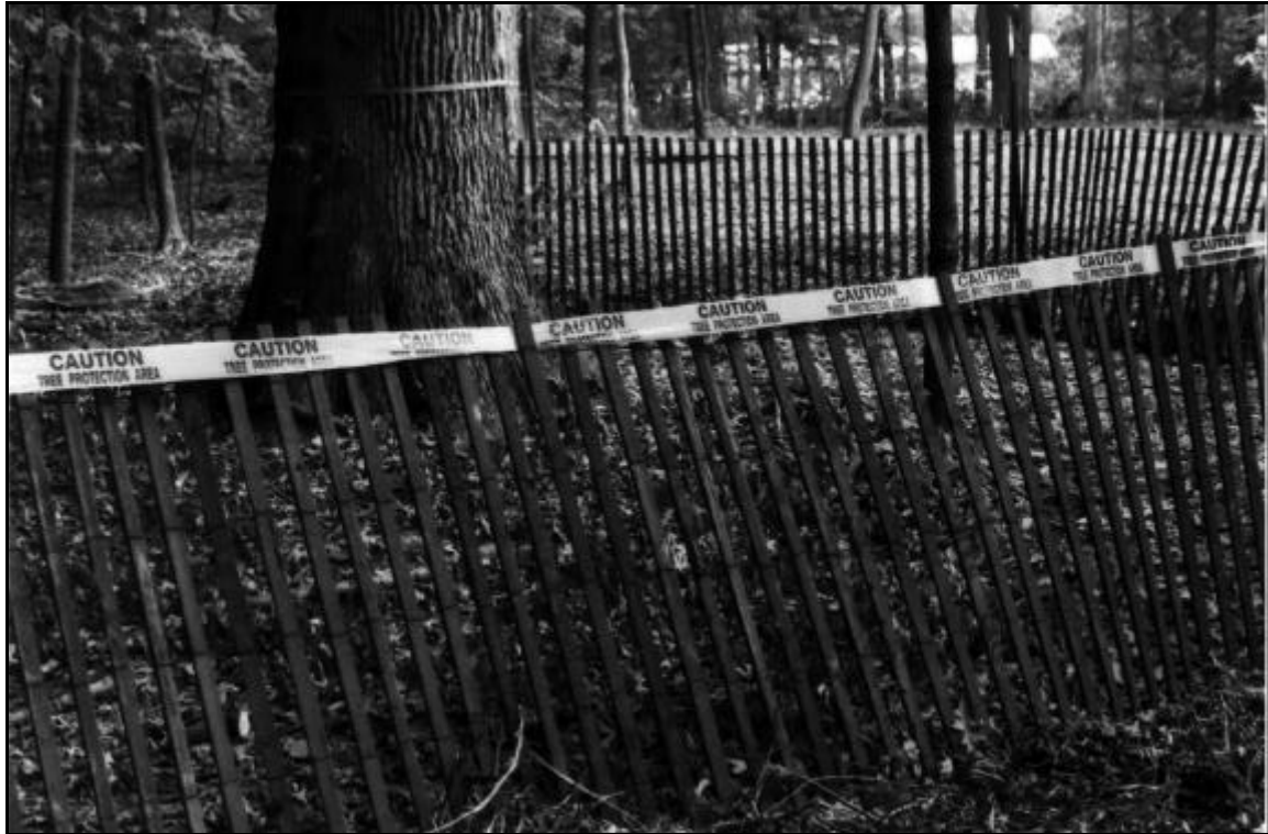
Exhibit 102a: Tree preservation and protection (Source: IDNR Files)
