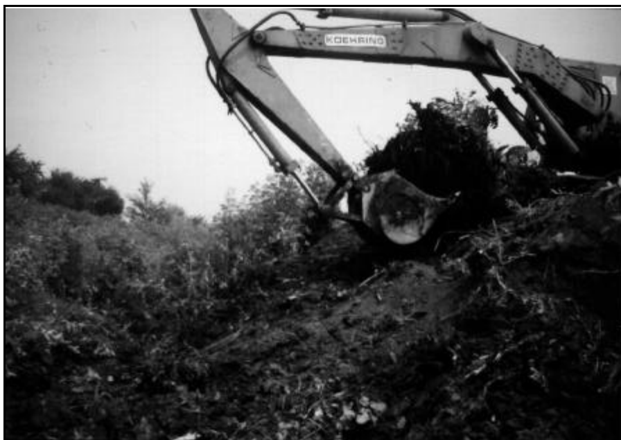
Exhibit 107a: Clearing and Grubbing (Source: NRCS Files)
