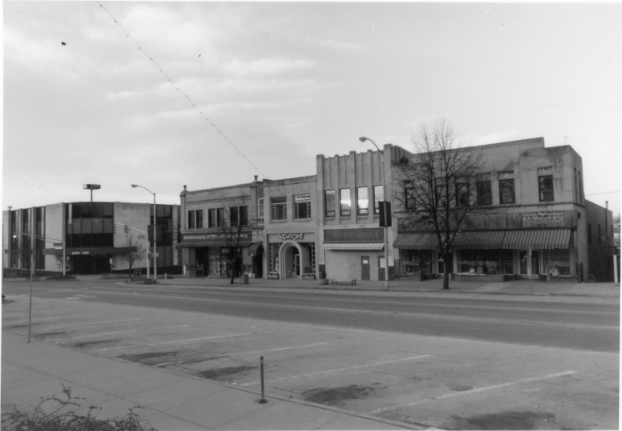
Figure 3: 107 and 109 N College from Courthouse Square Historic District National Register Nomination
