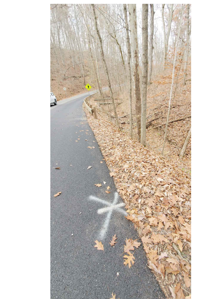
SITE 1 - EXISTING BANK (LOOKING WEST)
