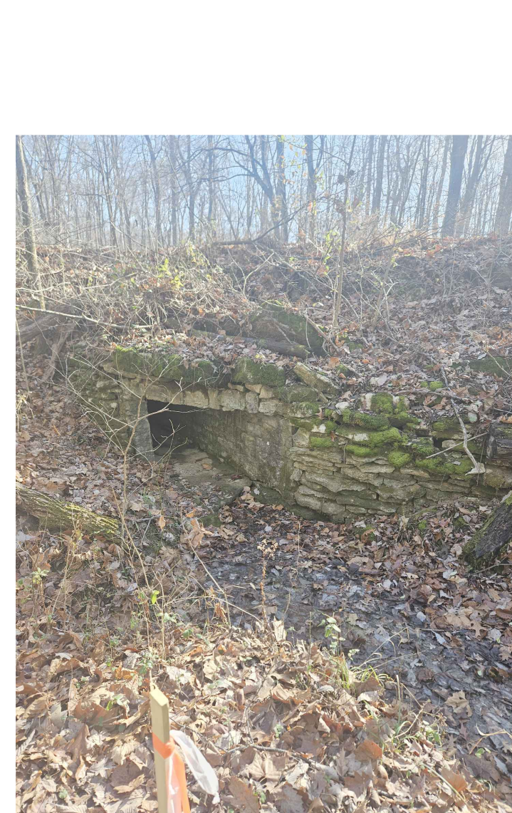
SITE 2 - DS END OF BOX CULVERT (LOOKING SOUTHEAST)
