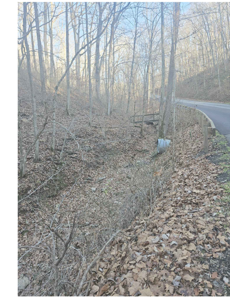
SITE 1 - DS END OF 48" CULVERT (LOOKING EAST)
