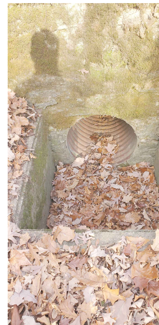
EXISTING 24" CMP HEADWALL/INLET
