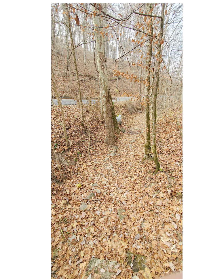
SITE 1 - EXISTING CHANNEL (LOOKING WEST)
