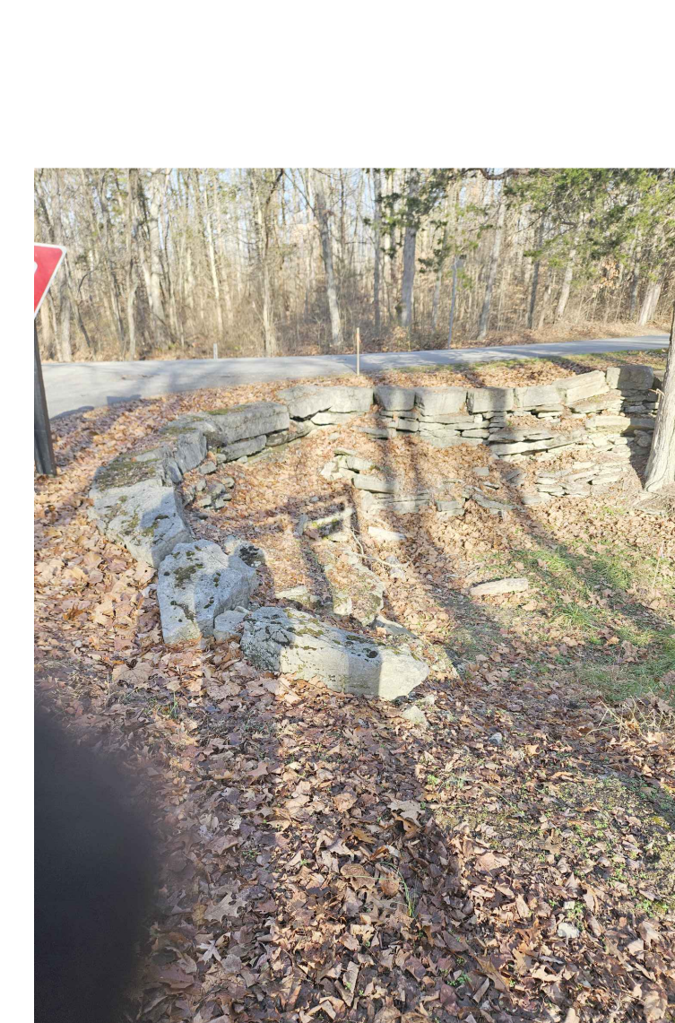
SITE 2 - US END OF BOX CULVERT (LOOKING NORTH)
