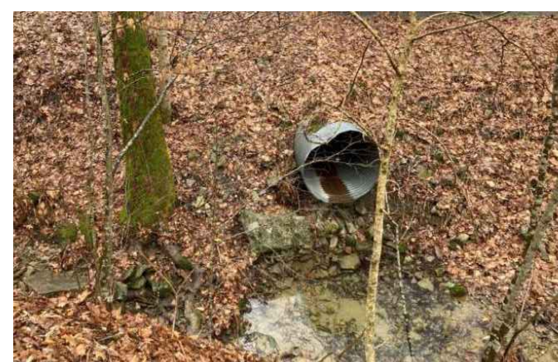
EXISTING 48" CMP OFFFALL
