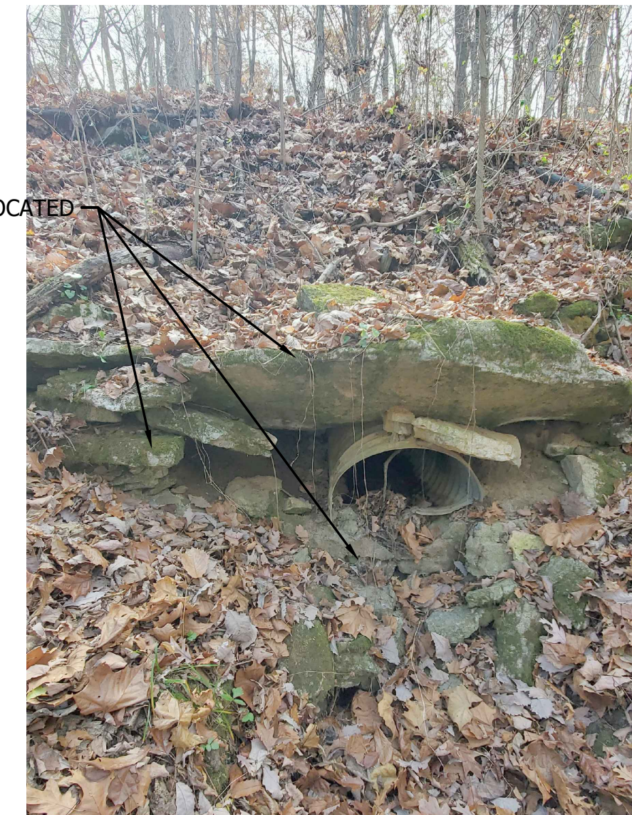
EXISTING 24" CMP OUTFALL
