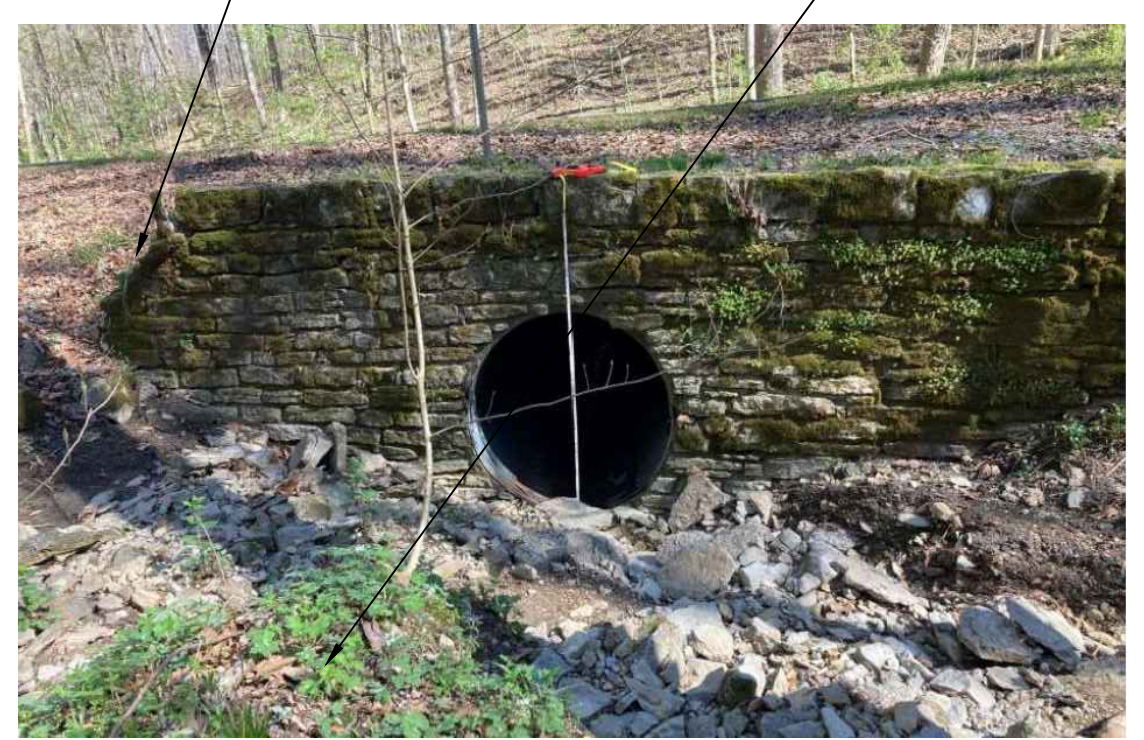
EXISTING 48" CMP HEADWALL/INLET
