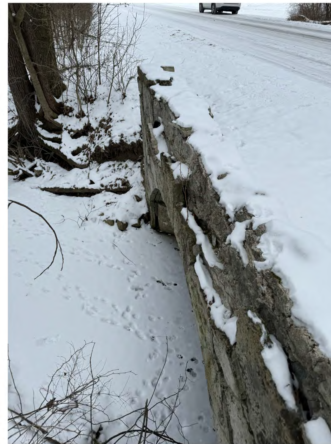
5. Side elevation at the upstream. Stone to be removed, salvaged, cleaned and reset.
