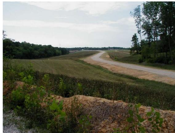
This project included the construction of a new ephemeral stream, a unique and diverse habitat that supports many plant and animal species. The 1,400 foot stream designed using natural stream morphology has a nonlinear shape and a variety of substrates. The stream should provide valuable wildlife habitat in addition to improving the water quality of Augusta Lake, which has persistent water quality problems associated with acid seeps.
