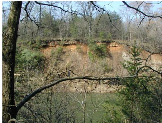
*Unconsolidated material at the top of the highwall would have continued to erode, undermining the surface stability.*
