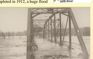
on the White River submerged the bridge deck under a few feet of water. The railings and decking were removed to prevent heavy debris from becoming entangled on the bridge. After the waters receded, the bridge was raised three feet higher and opened in 1913.
