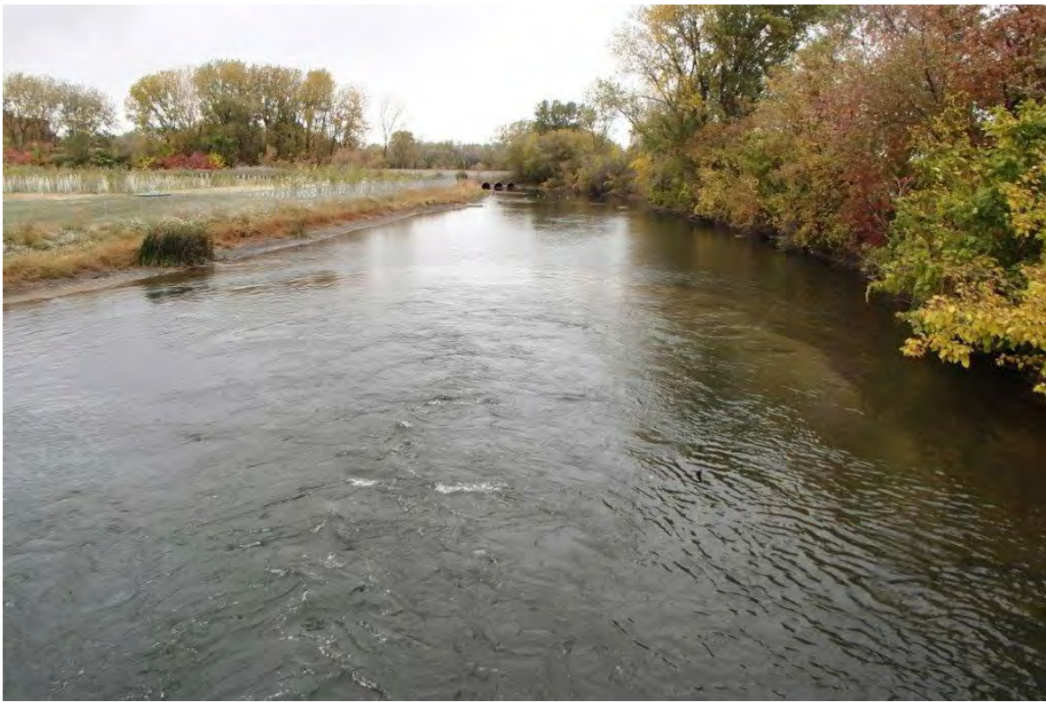
Grand Calumet River at the proposed NICTD crossing, from the Hohman Avenue Bridge, facing west.
