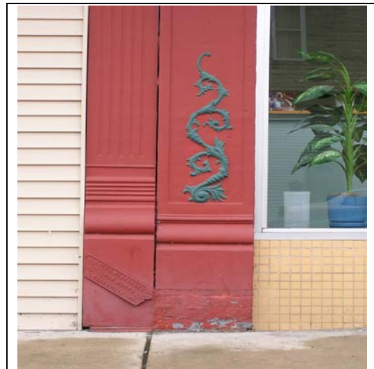
Cast iron storefront, Linton, Indiana. The nameplate on the left pilaster gives the name and city of the manufacturer. Some manufacturer's catalogs of cast iron architectural elements are still available. Photo by DHPA
