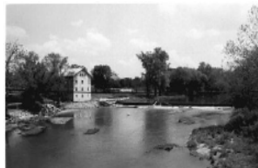
The Stockdale Mill in Wabash County. (Photo DHPA).
