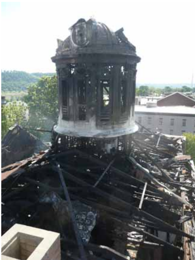
The cupola, roof and trusses of the Jefferson Co. courthouse after the May 20, 2009 fire. (Photo courtesy of Fritz Herget).
