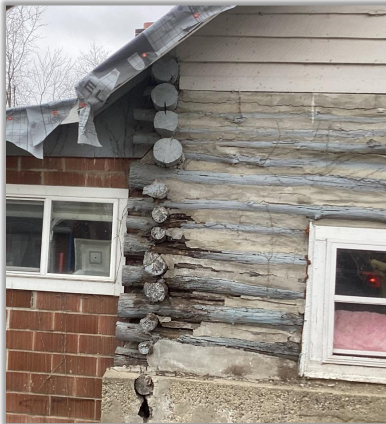
Above: Cabin in Bethany Park
