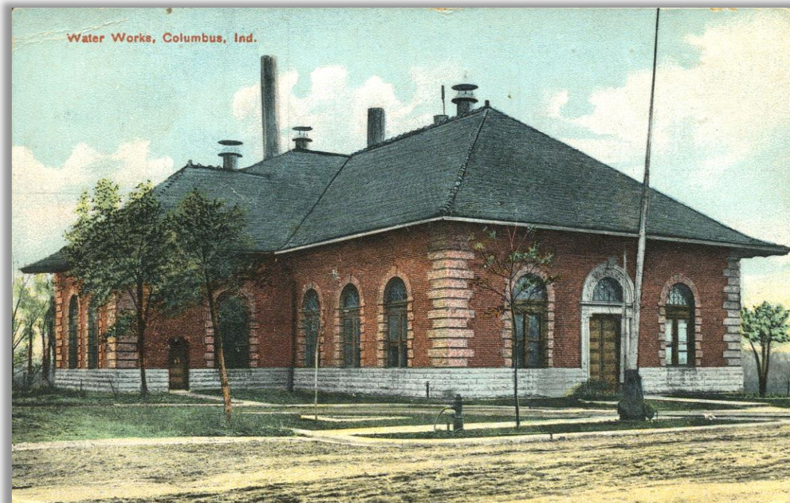
Above: Water Works, Columbus, Indiana, c. 1910, (From Indiana Album: John D. Rondot Collection)
