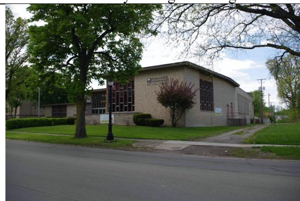
Camera facing southwest. The 1960 B'nai Jacob expansion (social hall/gymnasium) can be seen to the rear of the sanctuary. Photograph: Wendy Soltz, May 15, 2019.
