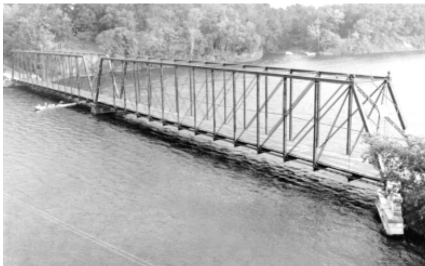
Tioga Bridge (1890) in White County, Indiana
