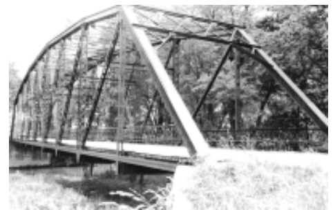
This 1916 Parker through truss was field-riveted, a tricky and unusual job for such a long truss.
