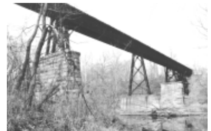
This plate girder viaduct is one of Indiana's longest and highest spans.
