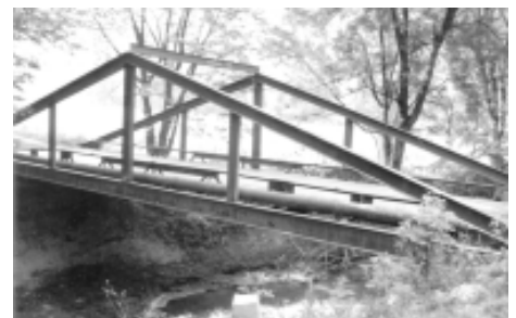
This Cantilever leg pony bridge was reinforced with a Kingpost arch, reducing the original trusses to little more than guardrails.
