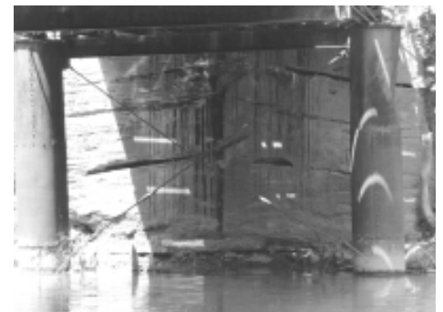
An example of metal caissons used to support an Indiana bridge.
