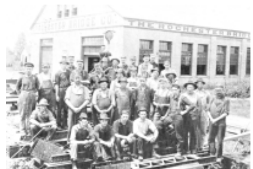
The staff and plant of the Rochester Bridge Company of Rochester, Indiana, circa 1910.
