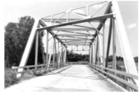
A 1935 Warren through truss built on a 36 degree skew.
