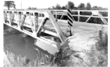
Two bridges from the same county: a 1900 Pratt pony (Above) and a 1917 Warren pony (below)
