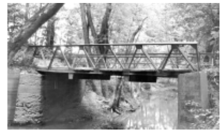
Some design variations: a Whipple hybrid (above) and a Warren pony/bedstead combination (below)
