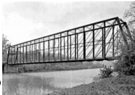
Laughery Creek Bridge (1878) in Dearborn County
