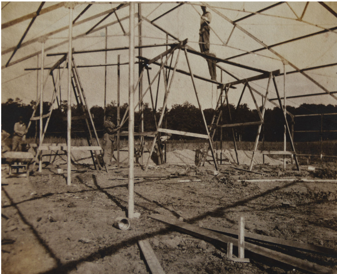
Figure 5. Greenhouse construction on the Peaper Farm, c. 1917. Peaper Family Collection.
