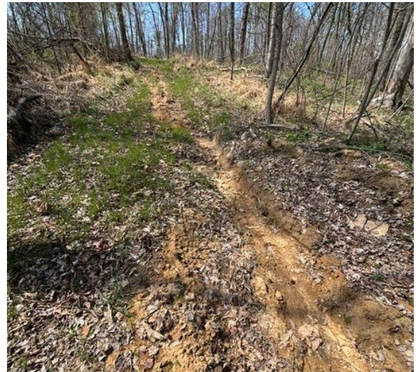
Heavy seeding and good revegetation can only protect the soil so much on a steep and long slope. Lack of water diversions on this skid trail is causing erosion and destabilizing the trail after a harvest. Photo by Jennifer Sobecki, DNR
