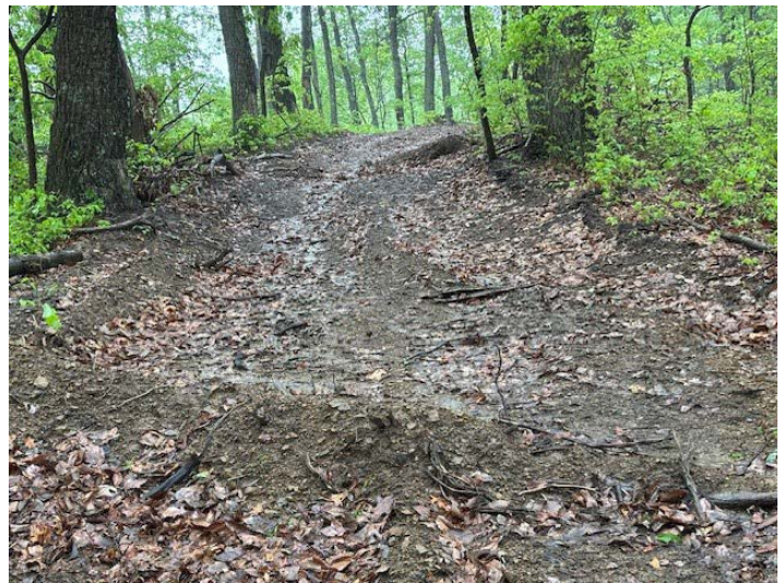
Top waterbar has been breached and water is flowing down the trail. The waterbar closest to camera is actively moving stormwater off a skid trail during a rain event. Photo taken on state forest lands by Jennifer Sobecki, DNR.
