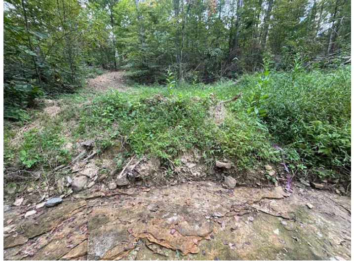
The waterbar before the crossing has revegetated well, but upon further inspection a breach has formed, allowing sediment laden runoff to enter directly from the skid trail in the stream after precipitation events (see purple tape on right side). Photo taken on state land by Jennifer Sobecki, DNR.
