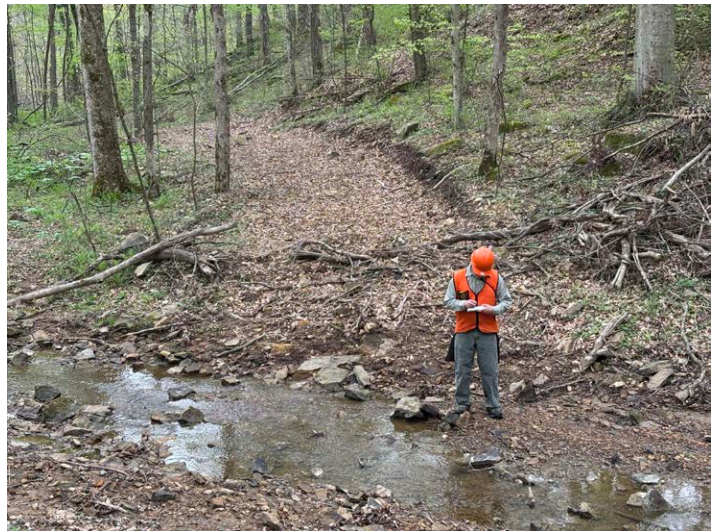
Good debris/soil waterbar prior to crossing is protecting water quality at this stream crossing. Photo taken on state forest property by Jennifer Sobecki, DNR.
