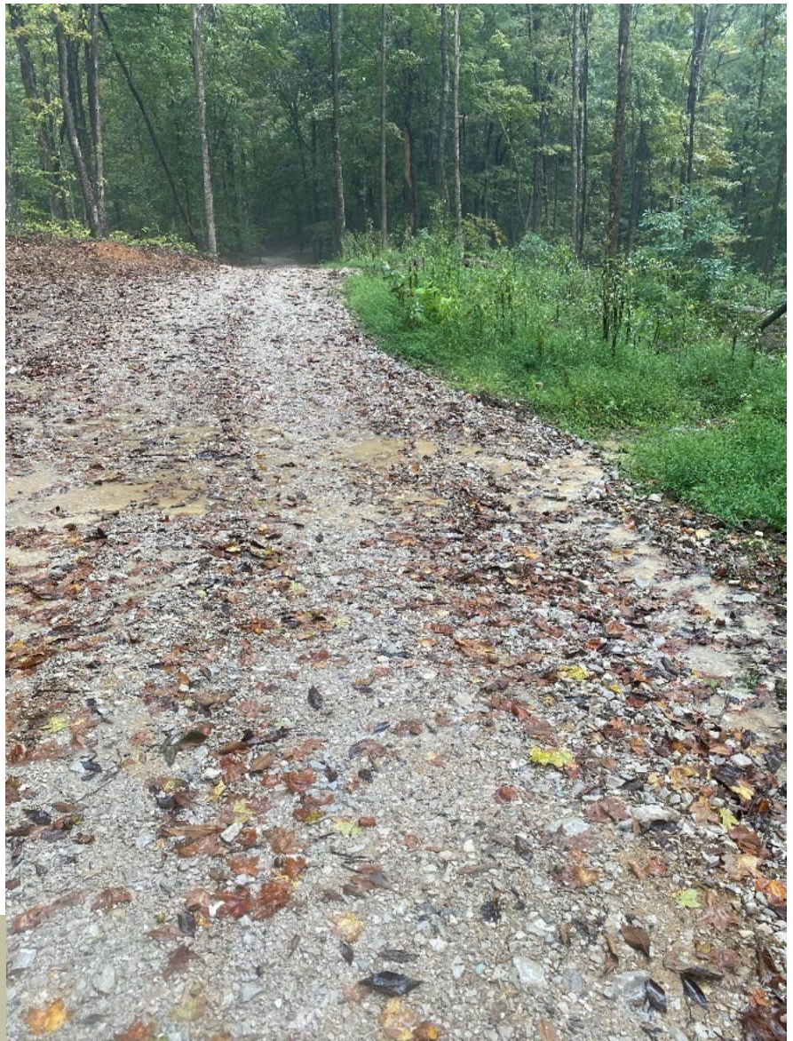
An outslope and cutout work to move runoff of an access road onto forest floor where it can be absorbed. Photo taken on state forest property by Duane McCoy DNR.
