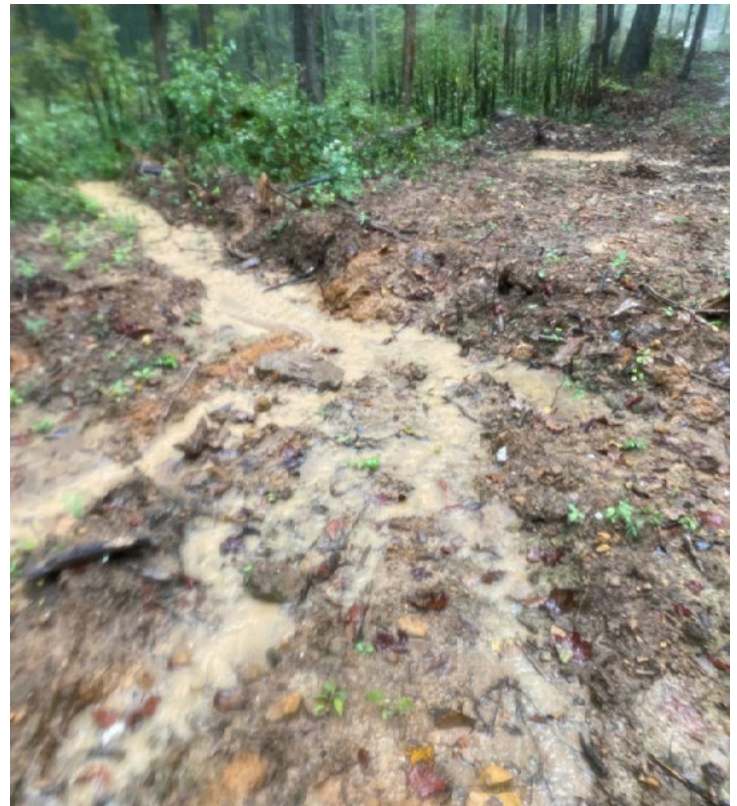
Waterbars actively moving stormwater off a skid trail during a rain event. Photo taken on state forest lands by Duane McCoy DNR.
