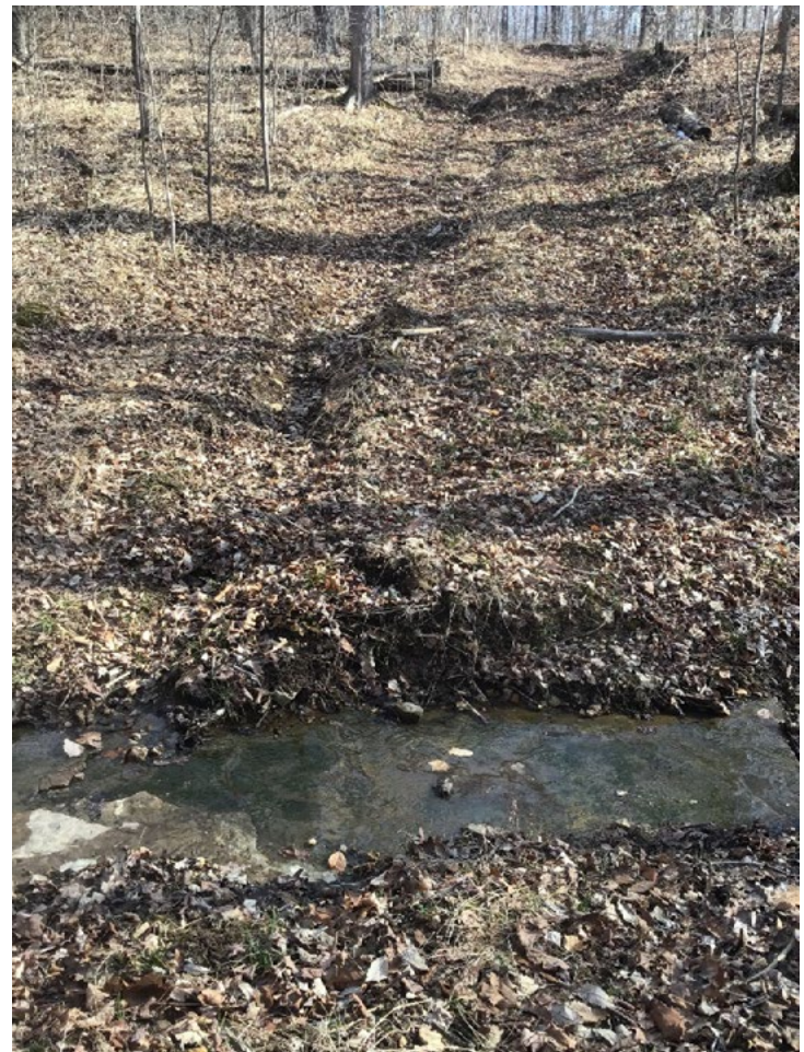
While there are waterbars leading down to the stream crossing, one more was needed before the crossing. Gully erosion is forming due to allowing the runoff to concentrate down the compacted trail and not diverting it before the crossing. Photo taken on private lands by Duane McCoy, DNR.
