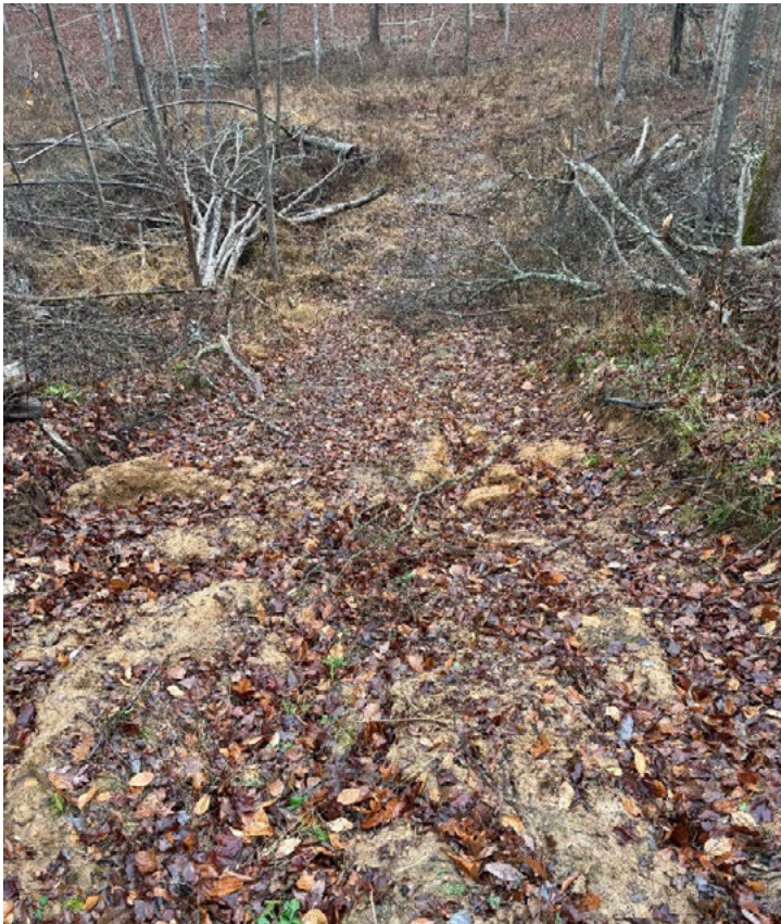
Blown waterbar above a stream crossing. Stream is filled with harvest debris. Photo taken on private land by Jennifer Sobecki, DNR.
