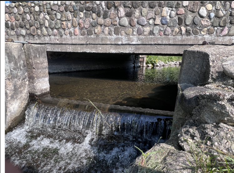
1. Side elevation Looking North. Some minor efflorescence visible along coping.
