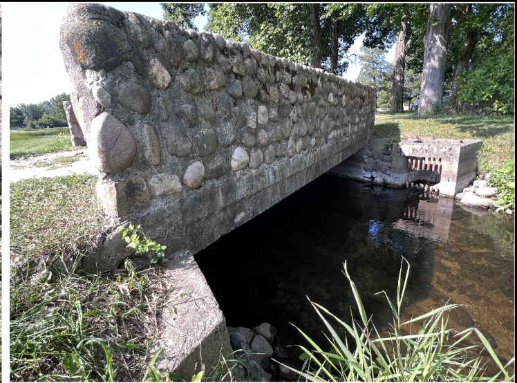
2. Looking West, efflorescence visible along deck coping. Some deteriorated mortar visible along end of abutment wall. Outside face of barrier wall visible, both barriers to be repaired by repointing.
