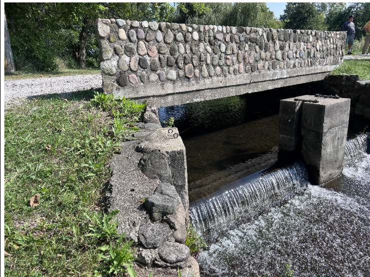
3. Side Elevation Looking North. Some minor efflorescence visible along deck coping. Outside face of barrier wall visible, both barriers to be repaired by repointing.
