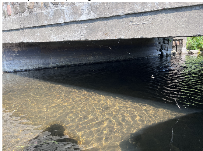
5. Looking west, afflorescence visible along deck coping. Some deteriorated mortar visible along length of abutment wall.
