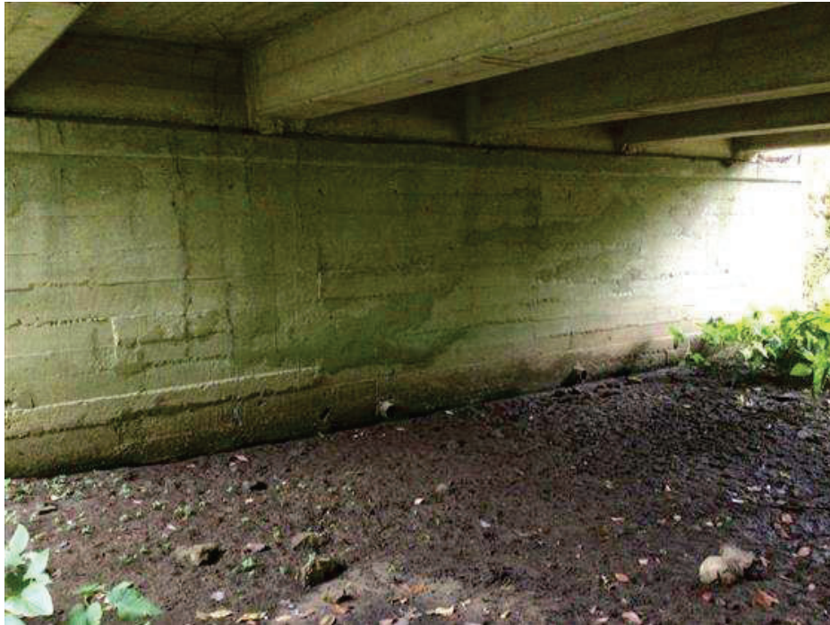
PHOTO 19 Condition Description Abutment 9
