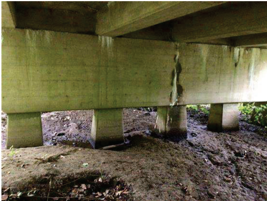
PHOTO 12 Condition Description Pier 5
