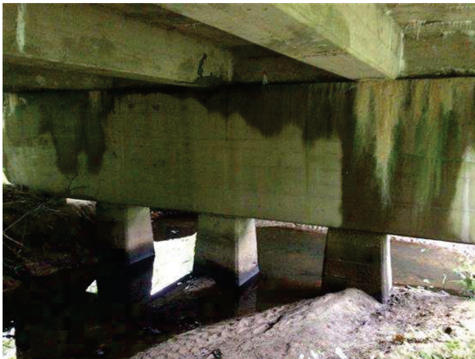
PHOTO 6 Condition Description Pier 3
