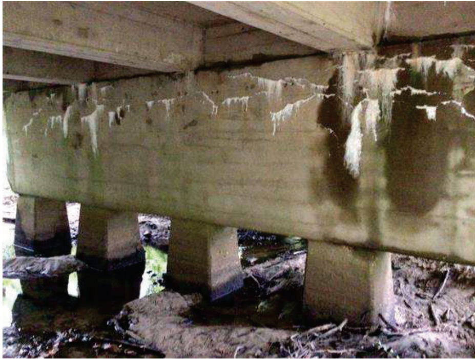
PHOTO 5 Condition Description Pier 2
