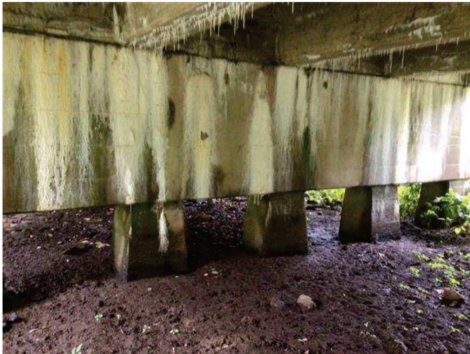
PHOTO 16 Condition Description Pier 7
