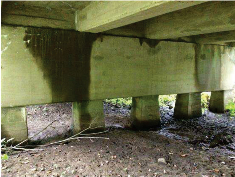
PHOTO 11 Condition Description Pier 6
