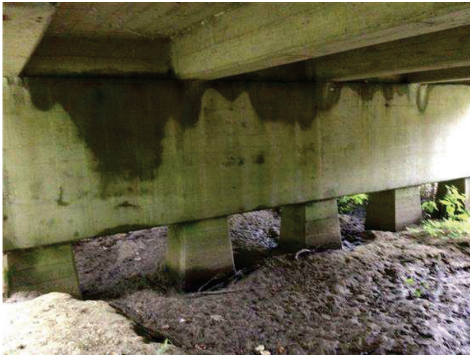
PHOTO 4 Condition Description Pier 4
