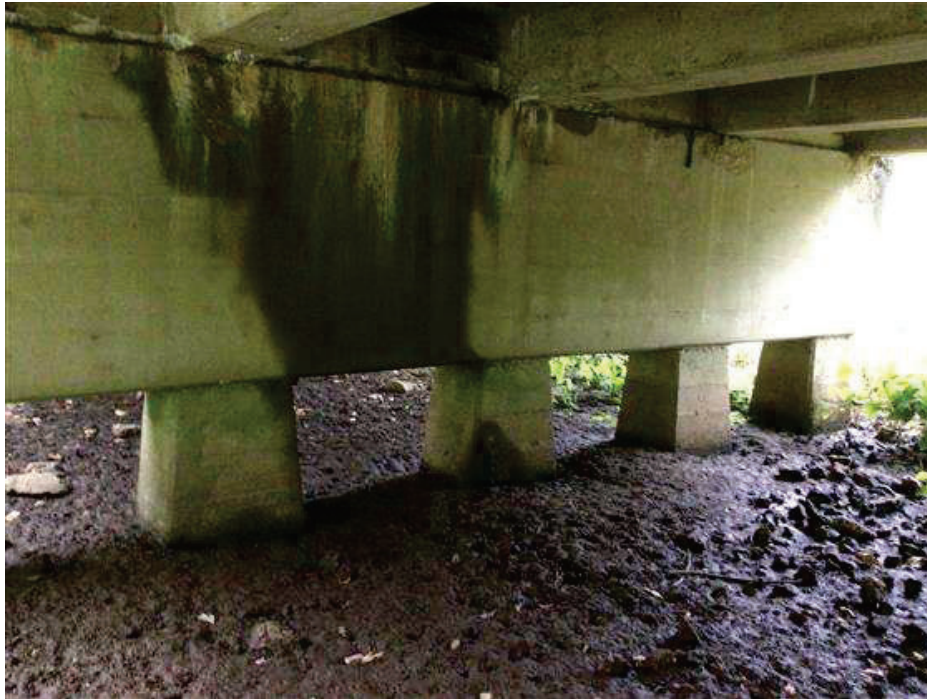
PHOTO 23 Condition Description Pier 8
