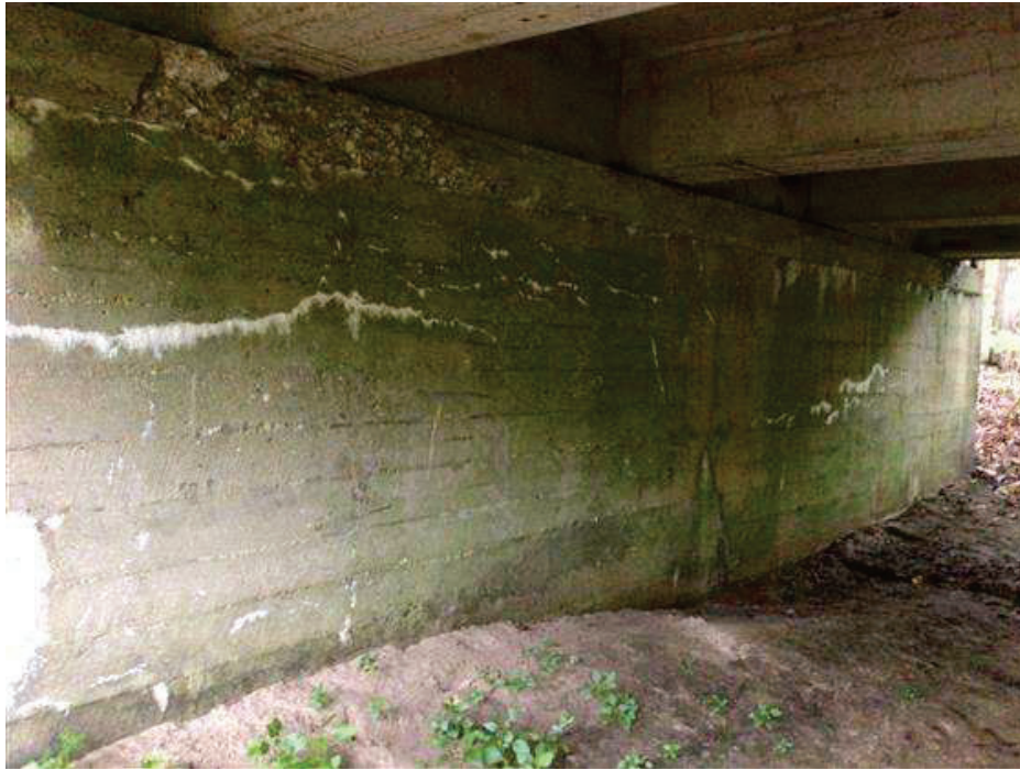
PHOTO 3 Condition Description Abutment 1 looking north
