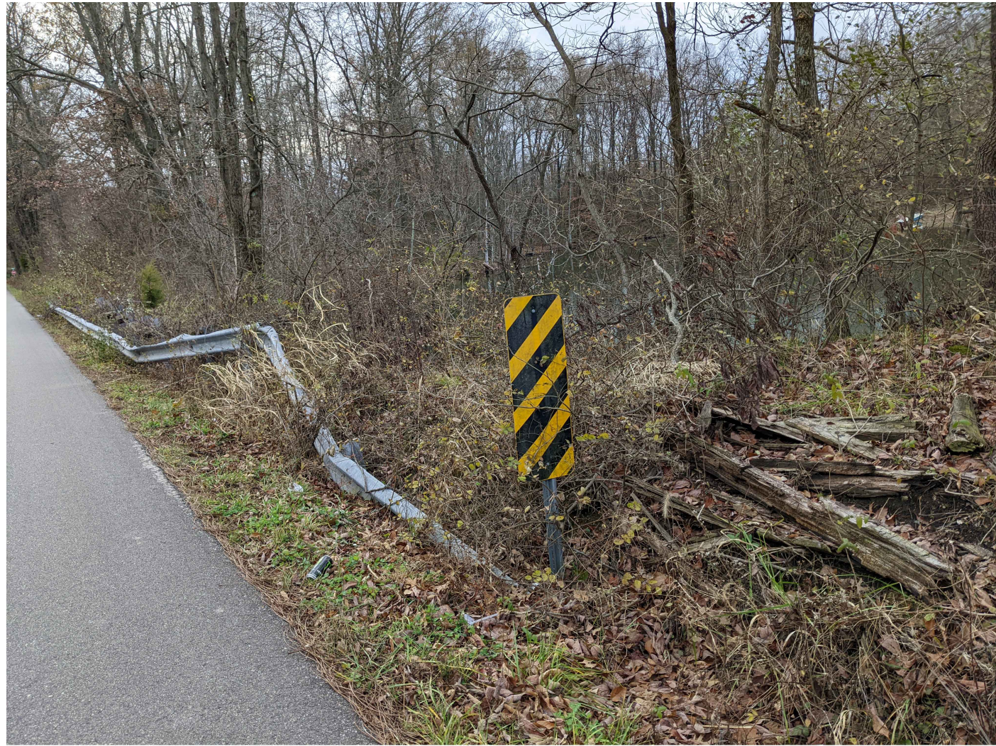
1 EX. DAMAGED GUARDRAIL WEST SIDE OF 12TH ST LOOKING SOUTH
