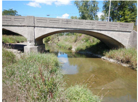
Photo 6: Project Bridge Facing North
