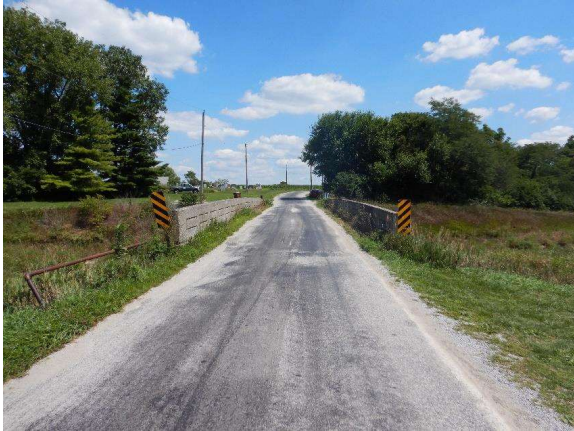
Photo 1: West Side Project Bridge Facing Southeast
