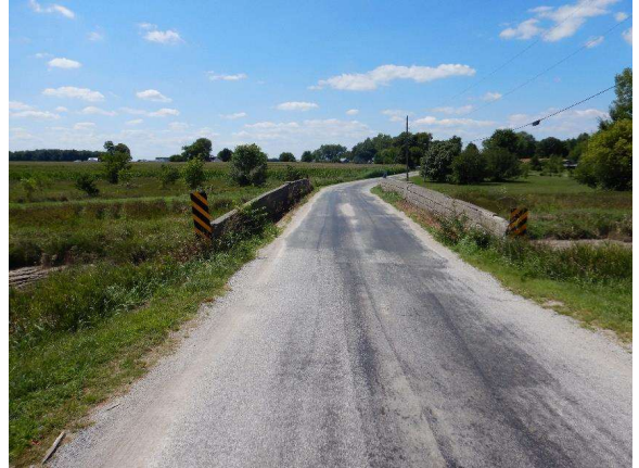
Photo 2: East Side Project Bridge Facing Northwest
