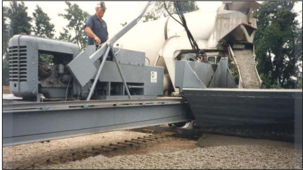
Figure 4-5. Concrete Spreader
