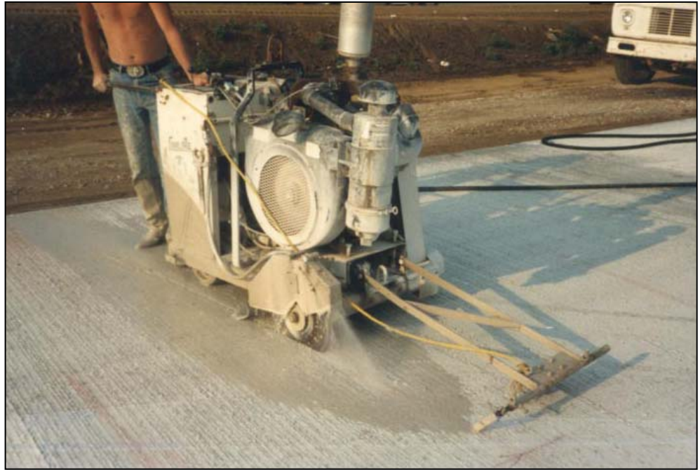
Figure 4-11. Self Propelled Concrete Saw
