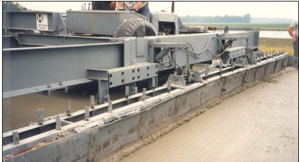
Figure 4-4. Finishing Machine
