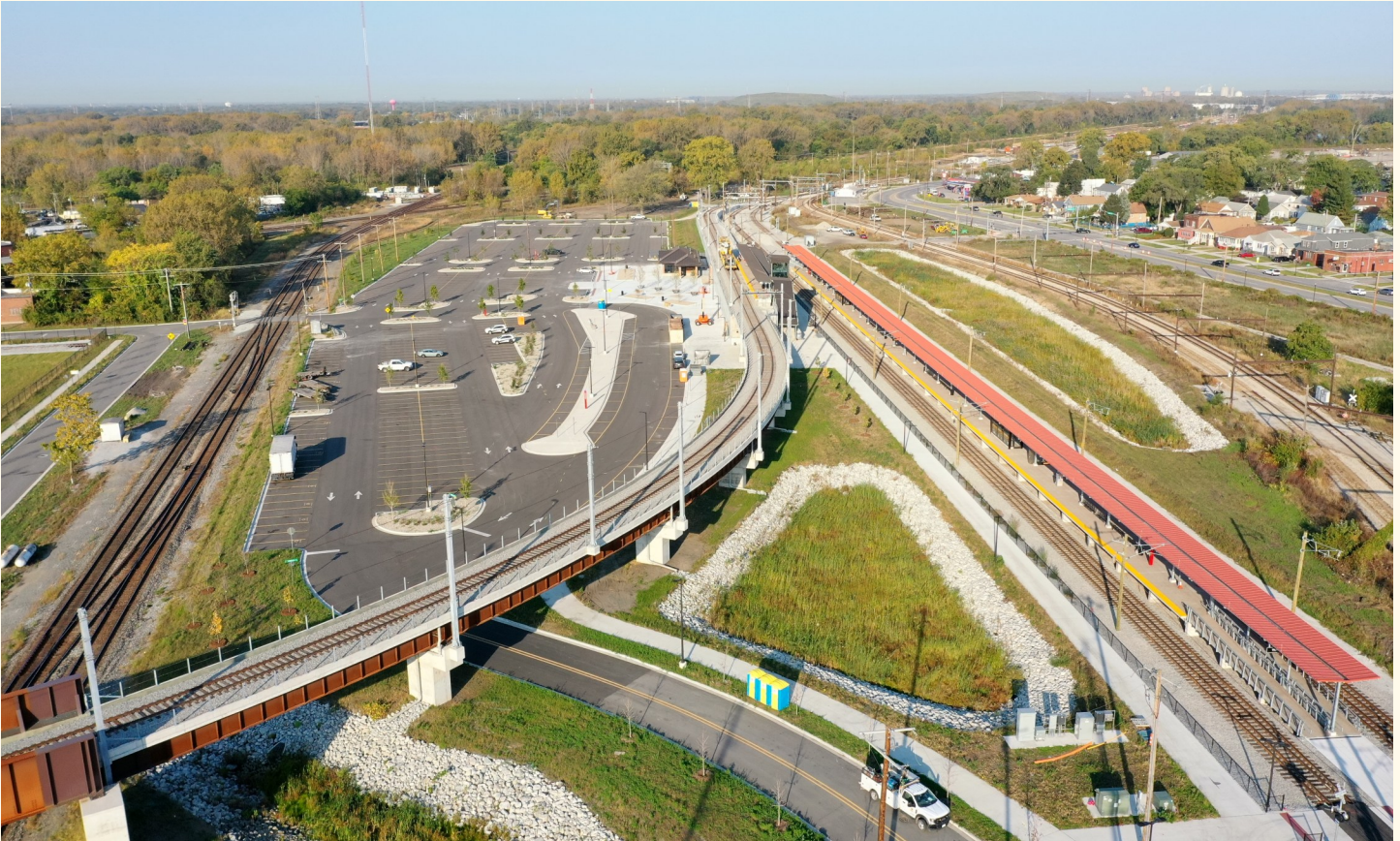
Gateway Station in Hammond seen as construction neared completion in 2024. The realigned main South Shore line can be seen coming in on the lower right, with the old alignment still present on the upper right. This will later be removed to provide land for Transit-Oriented Development. At left is the new West Lake, or Monon, line that runs south from here to the border of Munster and Dyer.
