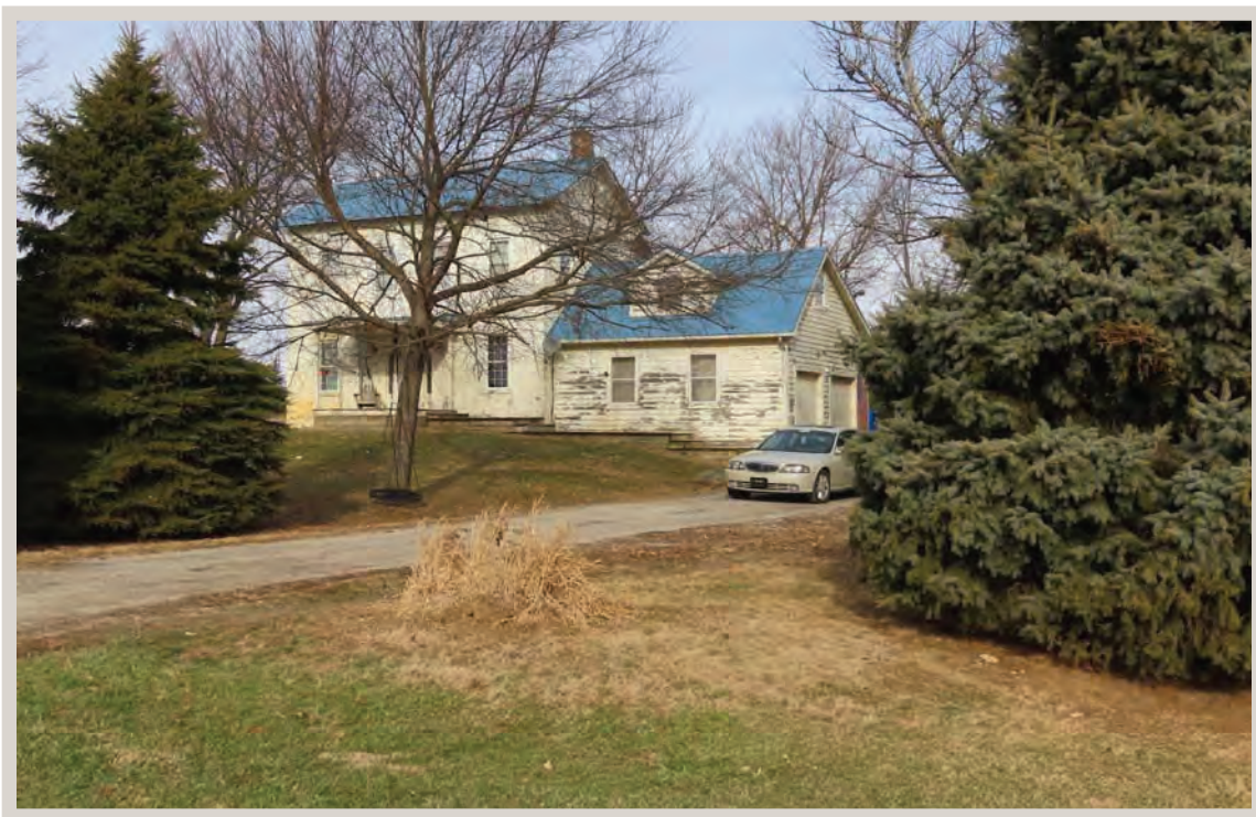
Looking northwest at the Endicott House from CR 600 South.
