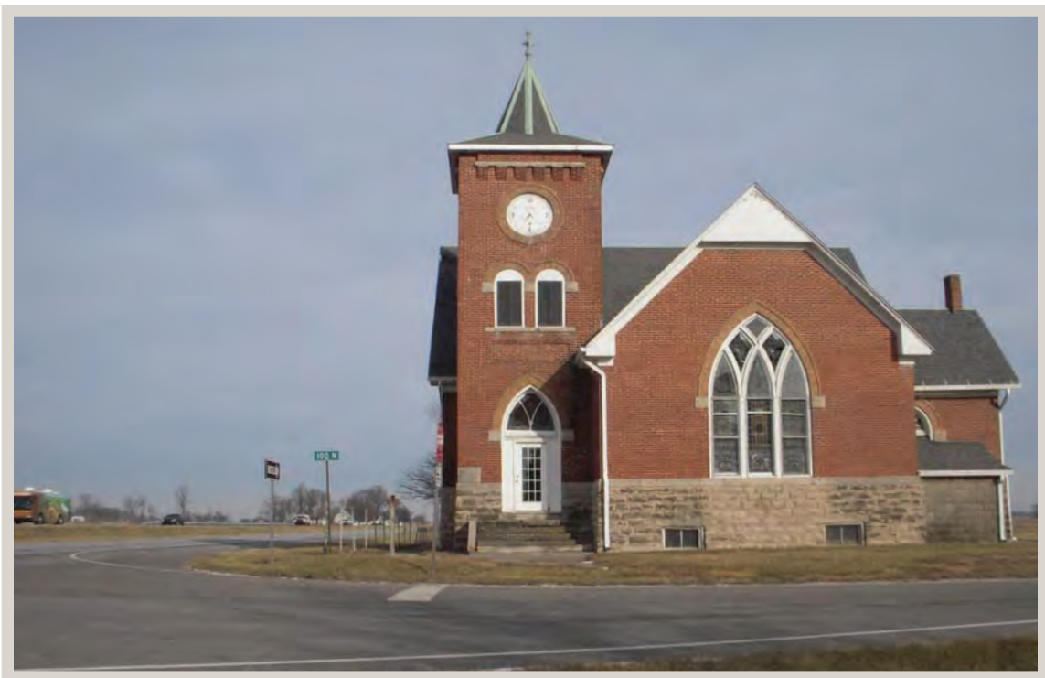
Looking north at Hopewell Methodist Church from the south side of CR 100 N.
