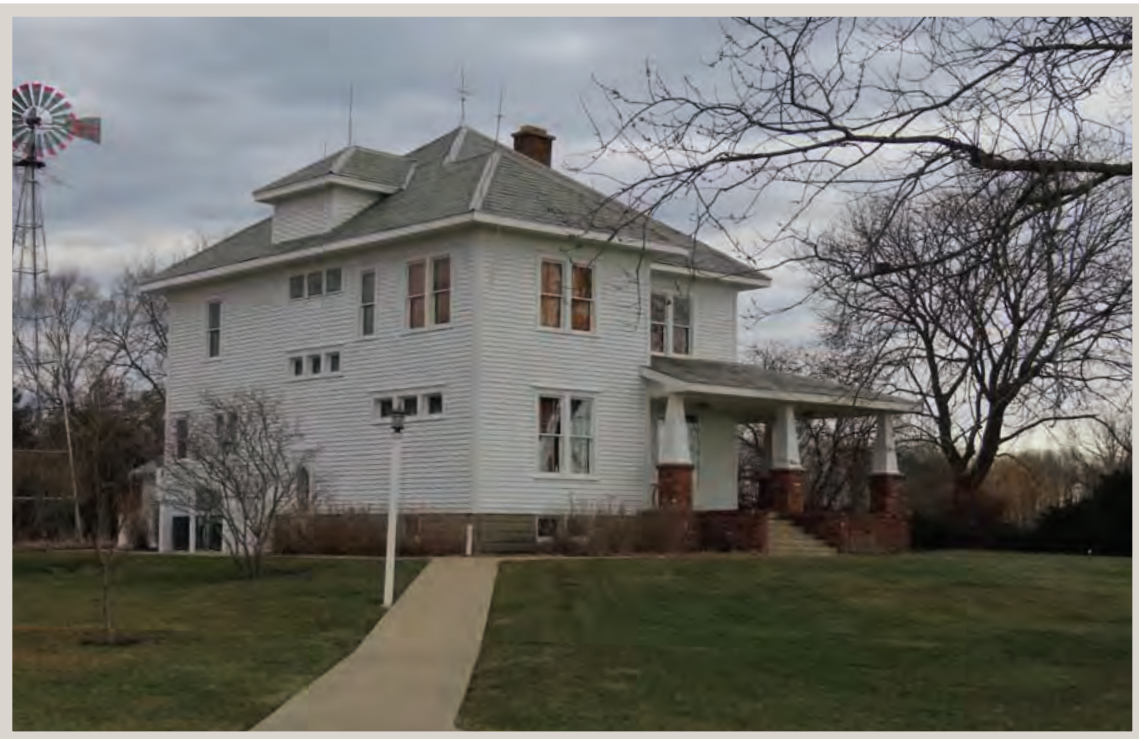
Looking northeast at the Kelley House. US 31 is beyond the trees at right.
