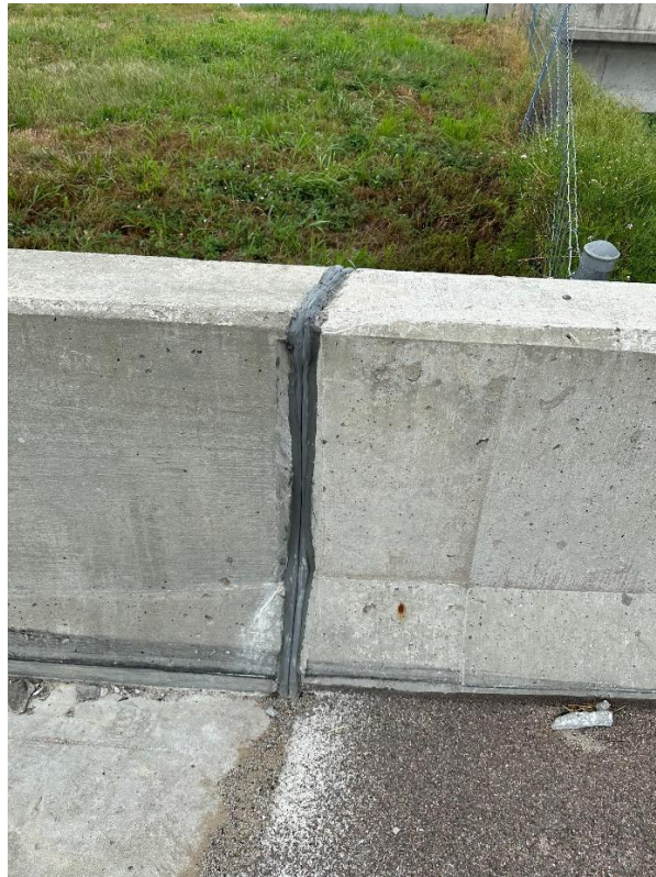
Figure 8: Pre-compressed foam sealer for bridge rail joints
