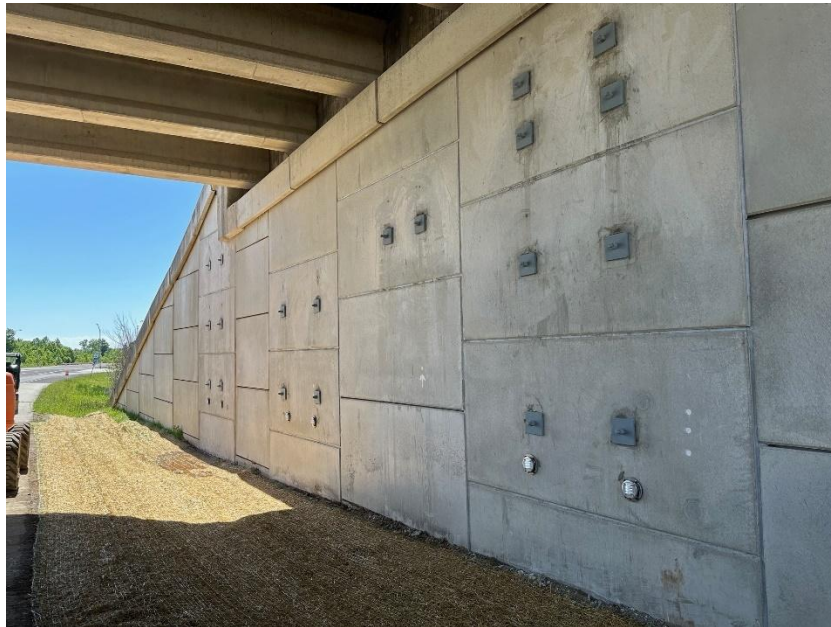
Figure 1: Rolled straw matting on the bench of the MSE wall
