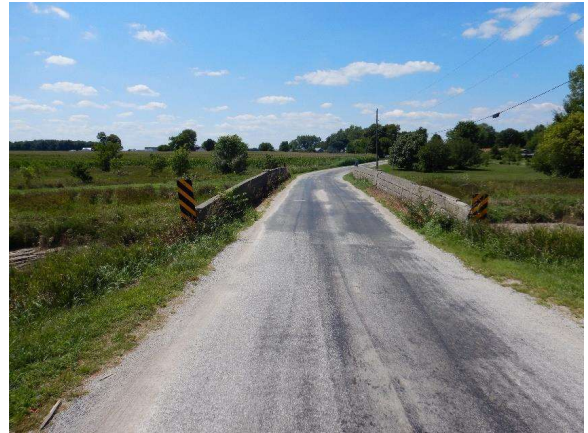
Photo 2: East side project bridge facing northwest
