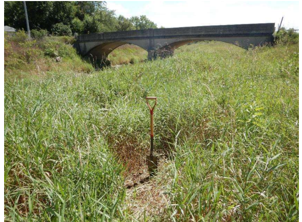
Photo 10: Sample Point 1 facing south towards project bridge
