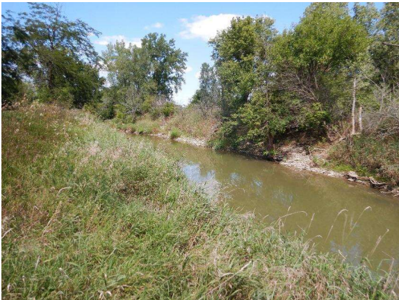
Photo 7: Rock Creek from north of project bridge facing northeast
