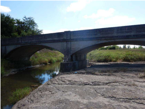
Photo 5: Project bridge and Rock Creek facing south
