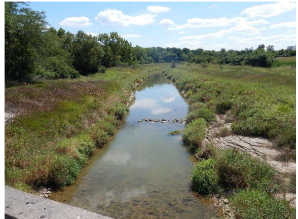
Photo 4: Rock Creek from project bridge facing south
