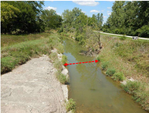
Photo 3: Rock Creek from project bridge facing north
