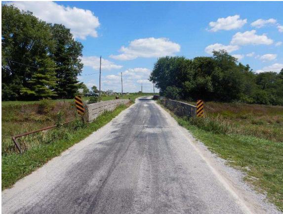
Photo 1: West side project bridge facing southeast
