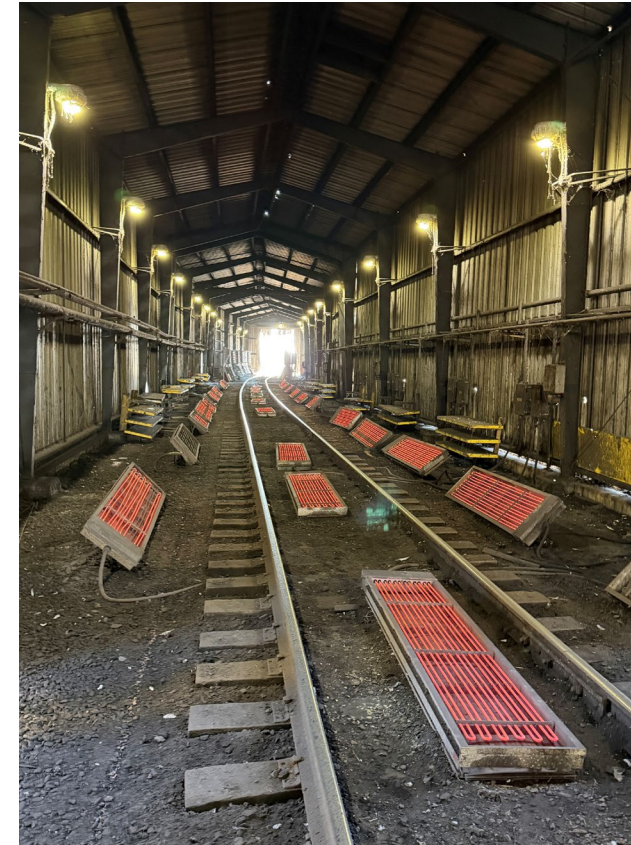
Gibson Station Coal Thaw Shed
