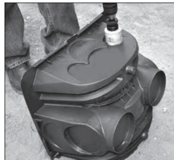
2. Drill pressure pipe hole.
