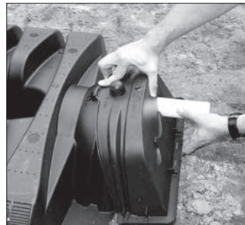
4. Place endcap over inlet end.
