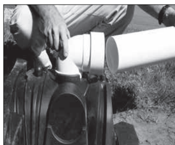
3. Connect inlet pipe.
