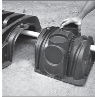
10. Lateral pipe through endcap.
