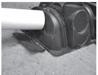
3. Insert inlet pipe.
