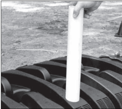
Chamber inspection port.
